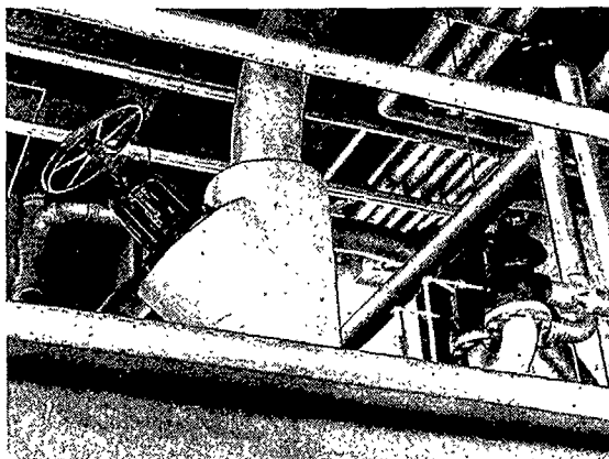
A stop-check valve on boiler lead to main steam header — in the boiler plant of large hospital.
