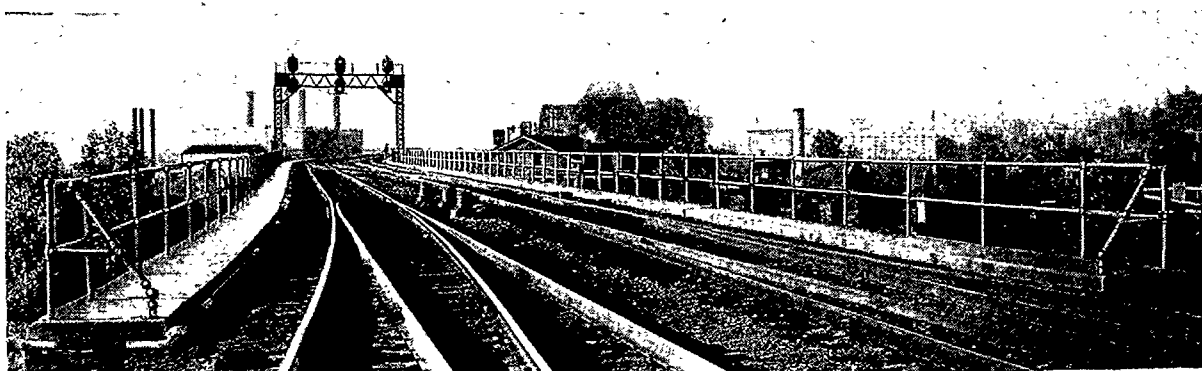
2-inch Galvanized Double Pipe Railing — total length of railing 6000 feet Fabricated in a Crane Branch House Shop
