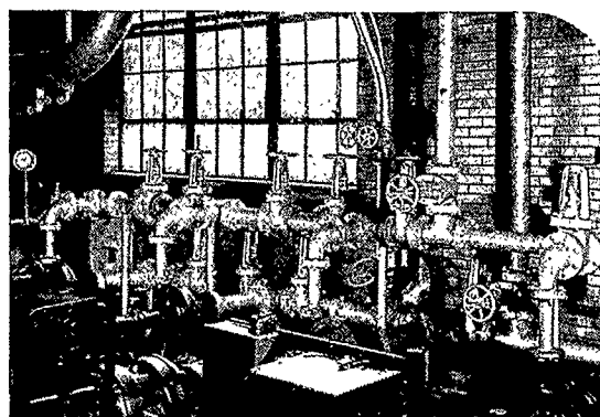
Crane iron valves and flanged fittings on the water circulating lines to coke ovens in a steel mill.
