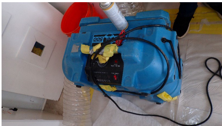
Figure 17: Air scrubber used in asbestos abatement. Air scrubber is used to filter out particulates before exhausting outside.
