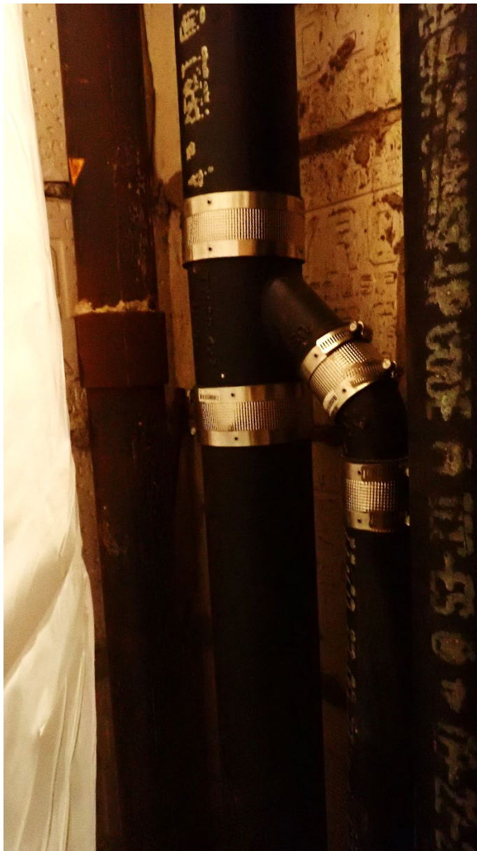
Figure 11: Pipe in wall cavity after asbestos abatement. Janitor Closet/Slop Sink, fourth floor.
