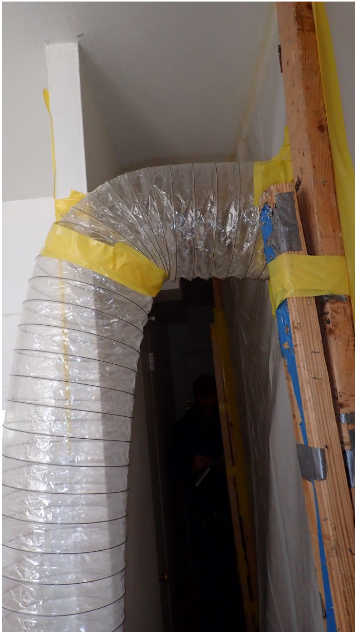
Figure 15: Outside edge of work area, and exhaust piping.
