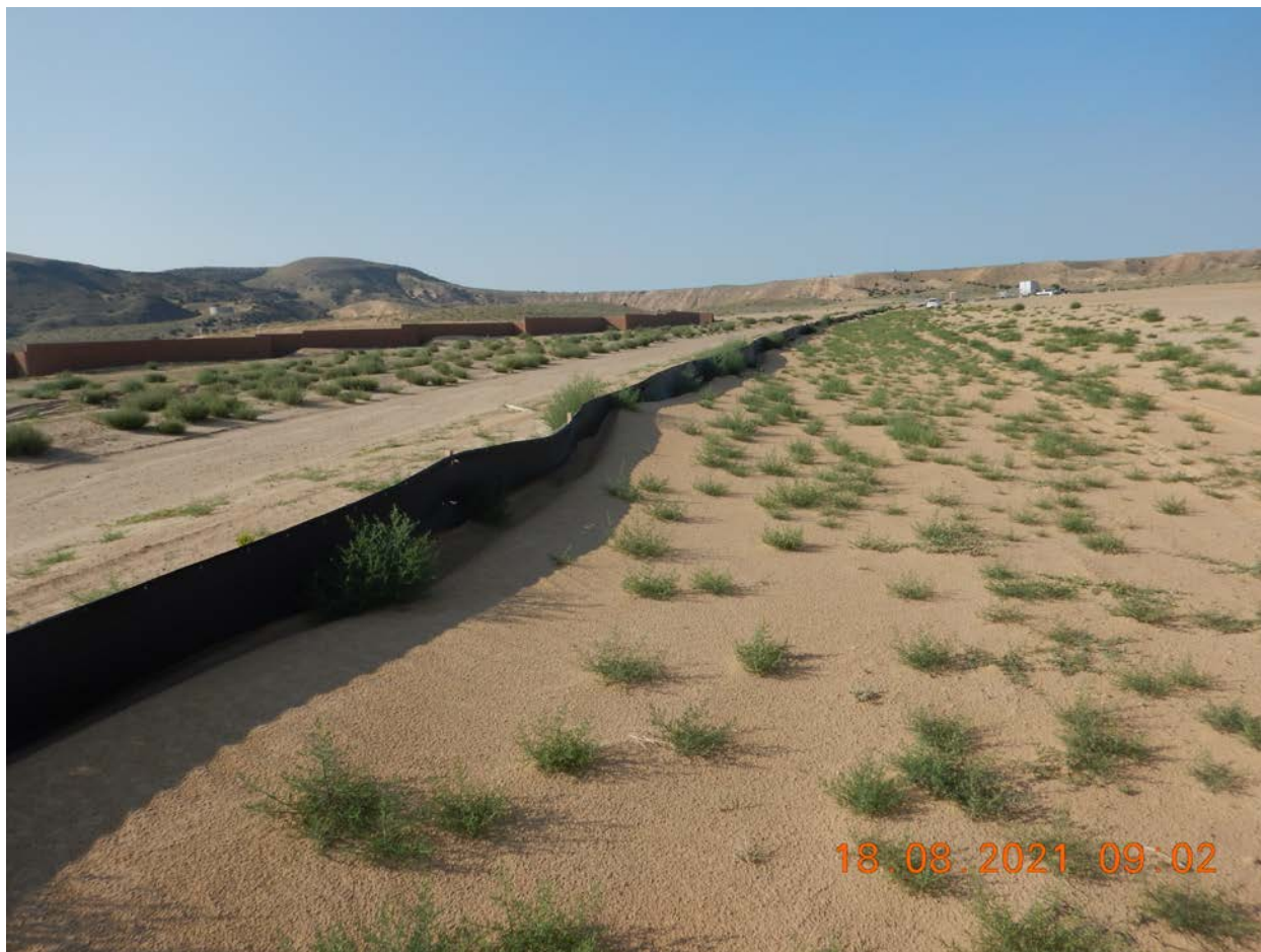
View looking approximately southwest towards Project trailer. August 18, 2021 (DSCN1939). Photographed by D. Esparza
