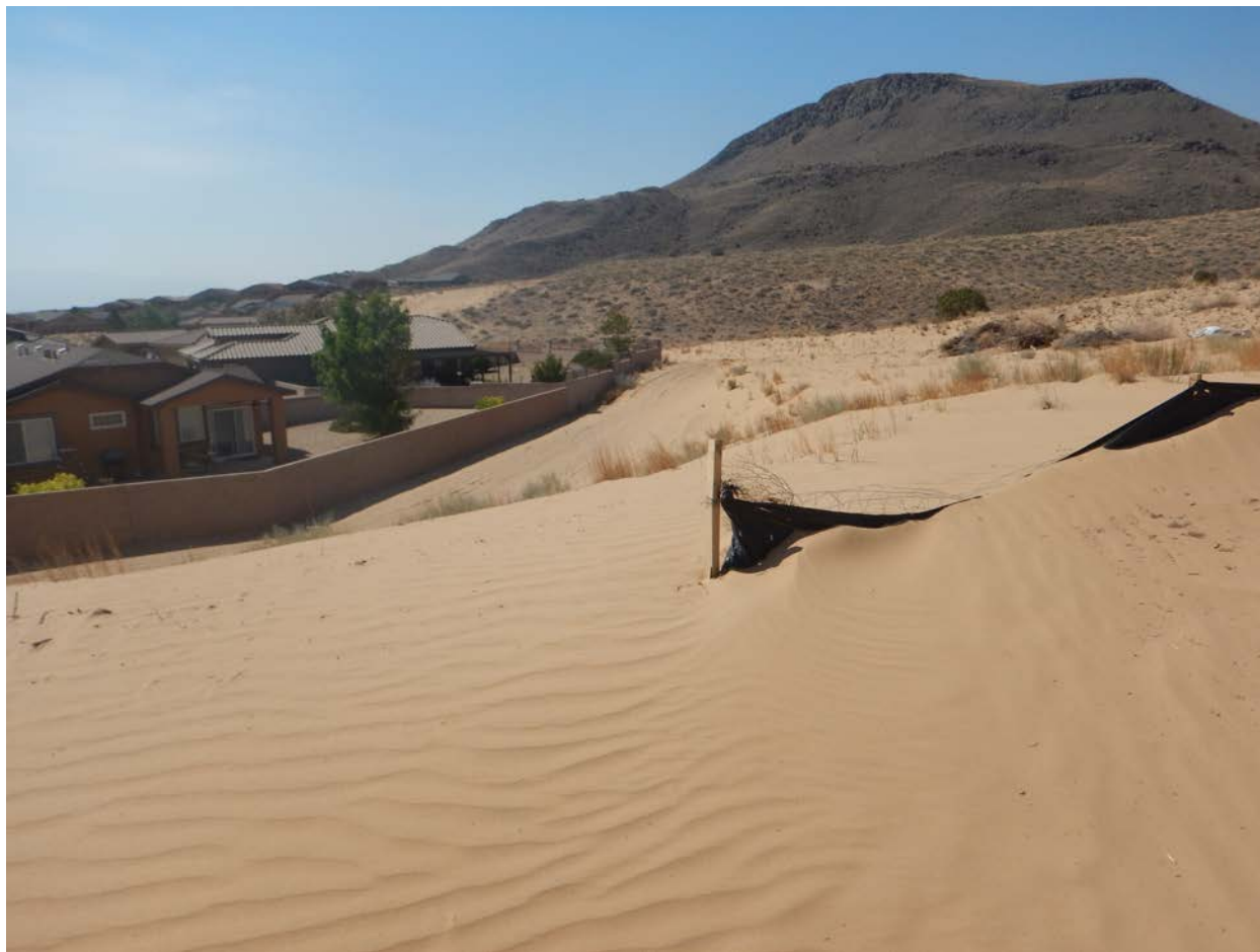
View of an accumulation of wind-blown overburden material and compromised silt fencing along Northside of Jubilee Subdivision. June 14, 2021 (DSCN1812) 10:11 AM Photographed by D. Esparza
