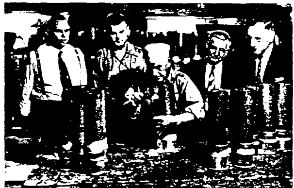
Left, an example of the type of plumbing used in the Darlington Apartments. All fixtures are connected to the soil lines with lead.
