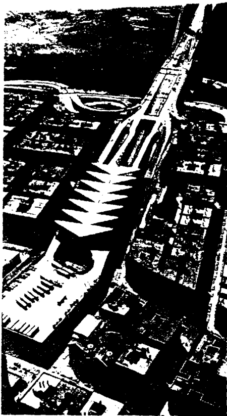
Aerial view of George Washington Bridge Bus Station looking west to the bridge and Hudson River Palisades.
