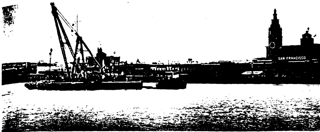
San Francisco Bound, a barge lays cables near one end of the route from Oakland across the Bay.
