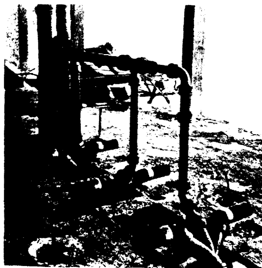
At the left, lead closet connections and lavatory wastes for a double toilet room, and at the right, similar roughing-in for the basement. All cast-iron joints were calked with lead
