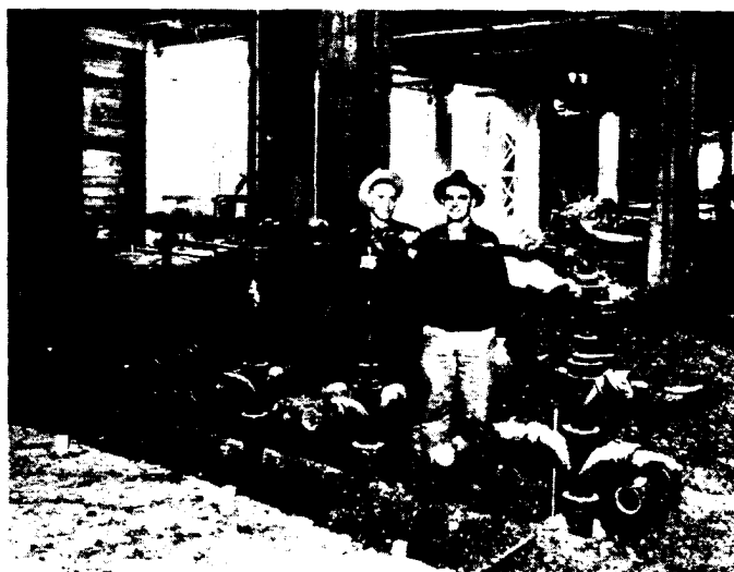
At the left, lead closet connections and lavatory wastes for a double toilet room, and at the right, similar roughing-in for the basement. All cast-iron joints were calked with lead
