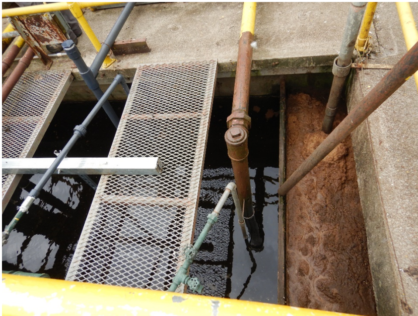
5: DSCN0183 Description: Clarifier Location: WWTP Camera Direction: ground Date/Time: 6/9/2021 11:12
