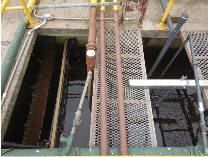
6: DSCN0184 Description: Clarifier Location: WWTP Camera Direction: ground Date/Time: 6/9/2021 11:48
