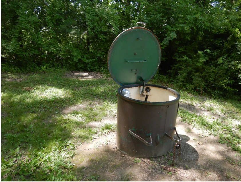
18: DSCN0196 Description: Aspen Lift Station Location: Camera Direction: Date/Time: 6/9/2021 14:33
