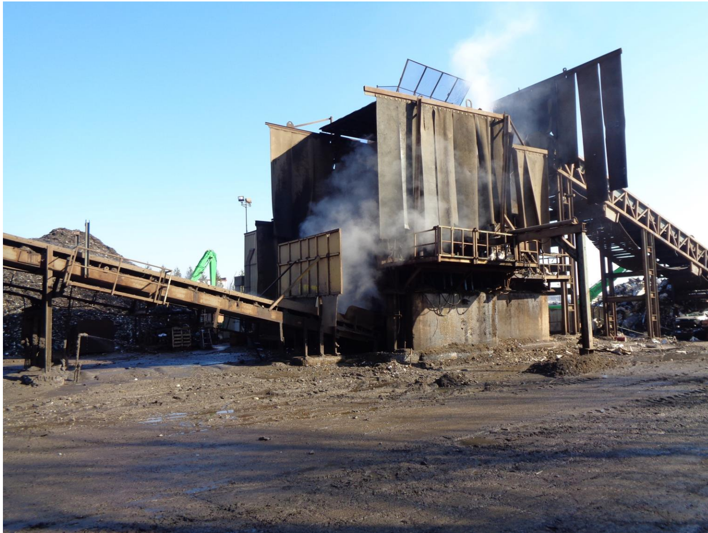
Shredder (back view) with conveyor to magnet sorting
