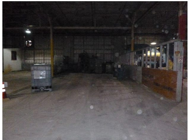
Photograph 4: Former Non-Hazardous Waste CAA.
