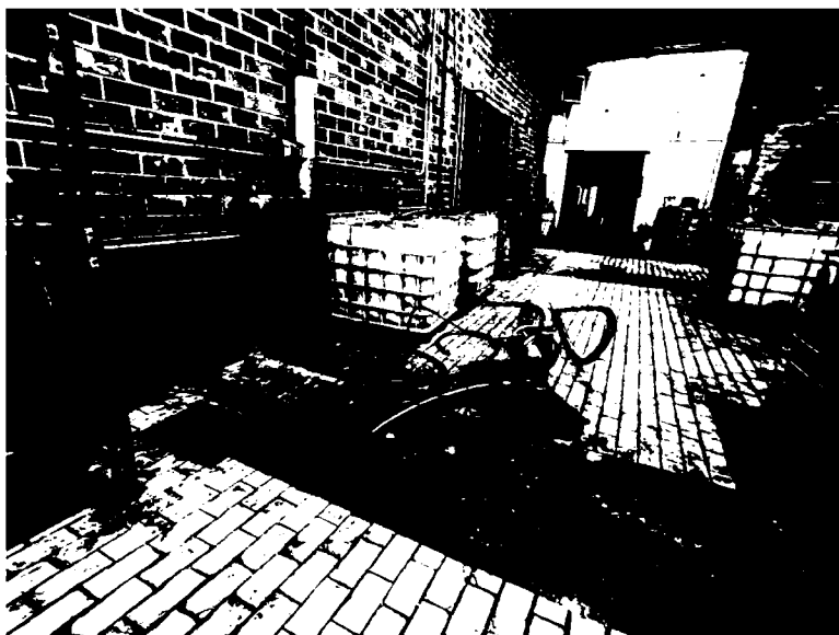
IMG_0469.JPG: Pump for pumping spills to a tote. Entire floor area is covered in residue from spills and chemicals puddles on the floor and evidence of acid etching of cement flooring.
