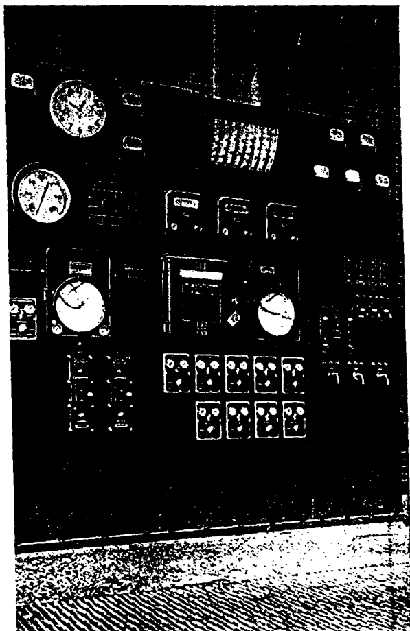
Fig. 3—Boiler room instrument panel
