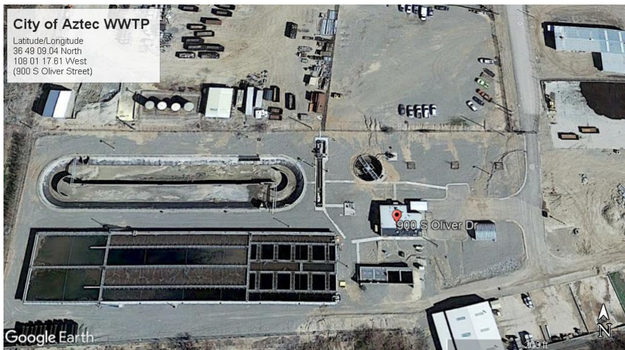
Aerial Image #1 Overall view of the City of Aztec's Wastewater Treatment Plant. Aerial from Google Earth.
