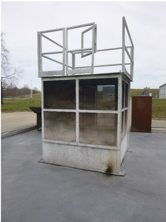
Photo 3: RCRA Permitted Pellet Treatment Unit
