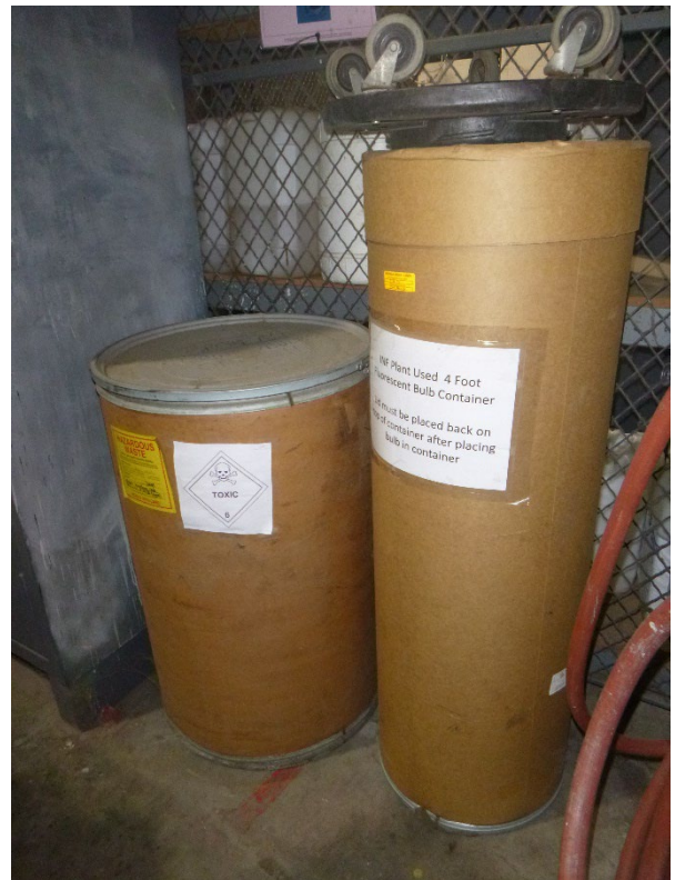
Photo 22: Hazardous Waste and Universal Waste lamp containers.
