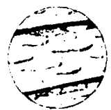
THIS IS BLISTERING
