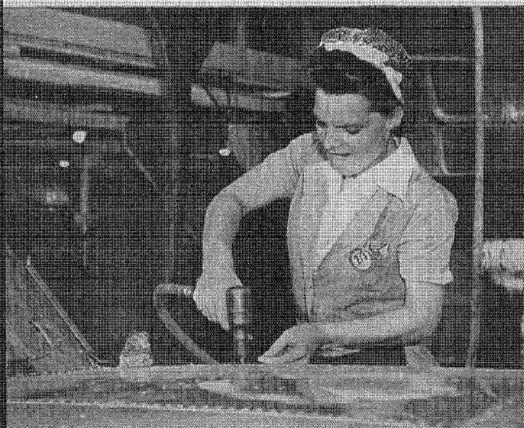
In cellophane the rivets stay cold for an hour or even longer, calling for fewer steps for this busy young lady
