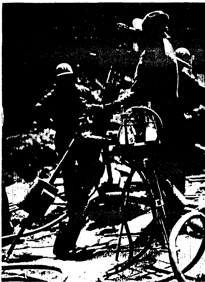
ROCK DRILL MOUNTED ON TRIPOD AND EQUIPPED WITH DEVICE FOR THE ELIMINATION OF SILICA DUST (The bottles shown on the tripod measure the amount of silica which will be inhaled by the drill operator.)
