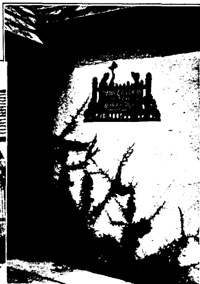
Silhouette shingle made from antimonial sheet lead, on an architect's office in Seattle.
