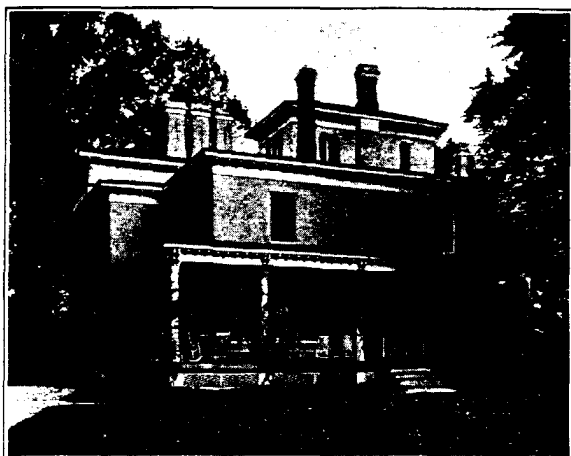
The stucco walls of the Von Kapff house at Stoneley, Md. were painted eight years ago with pure white lead, and the paint is still in excellent shape.
