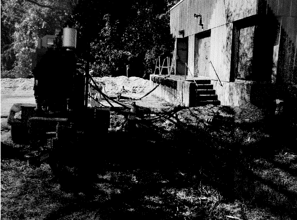
Photo 2 – Screen Building Pump
