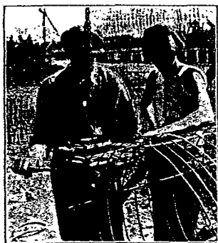
Cases being welded by Allan Portable Welding Machine
