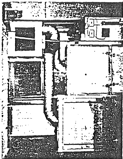
FIG. 3. Outflow end of two boxes showing connections to exhaust system.
