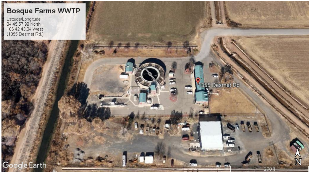
Aerial Image #1- Overall view of the Village of Bosque Farms Wastewater Treatment Plant. Aerial from Google Earth.
