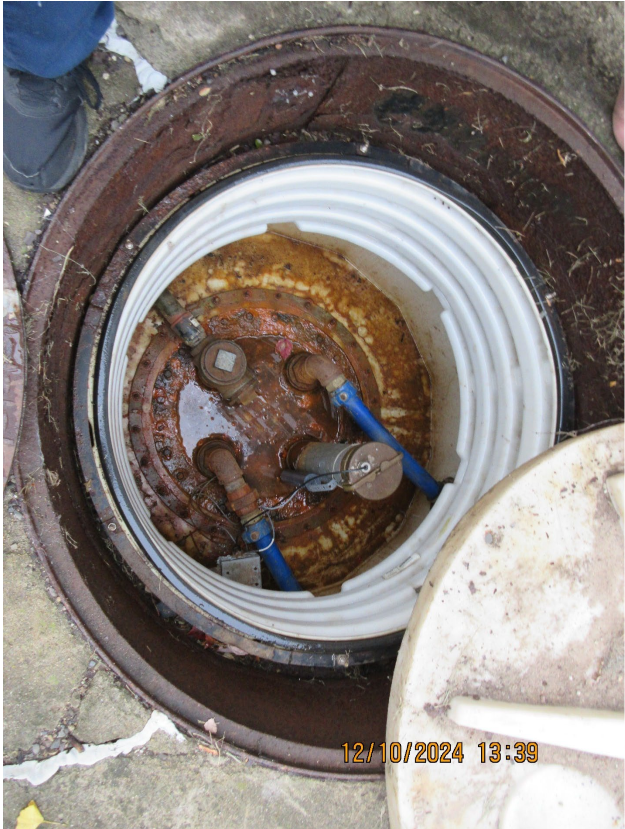
Photo 8 – Another angle of the interior of the turbine sump.
