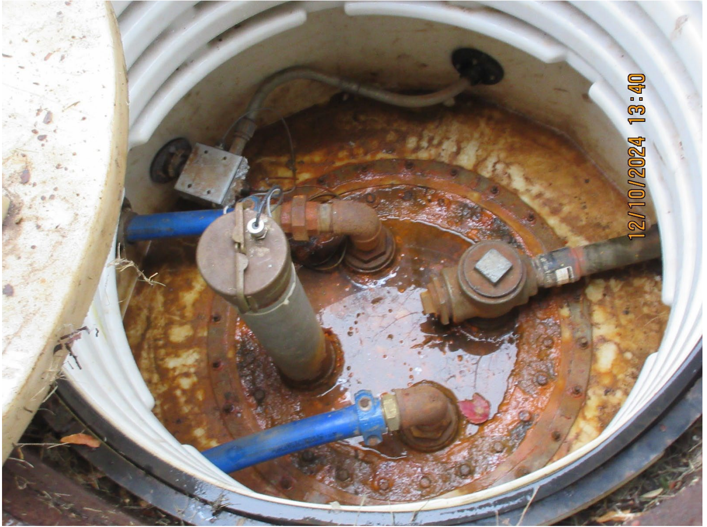
Photo 7 – Interior photograph of the turbine sump.
