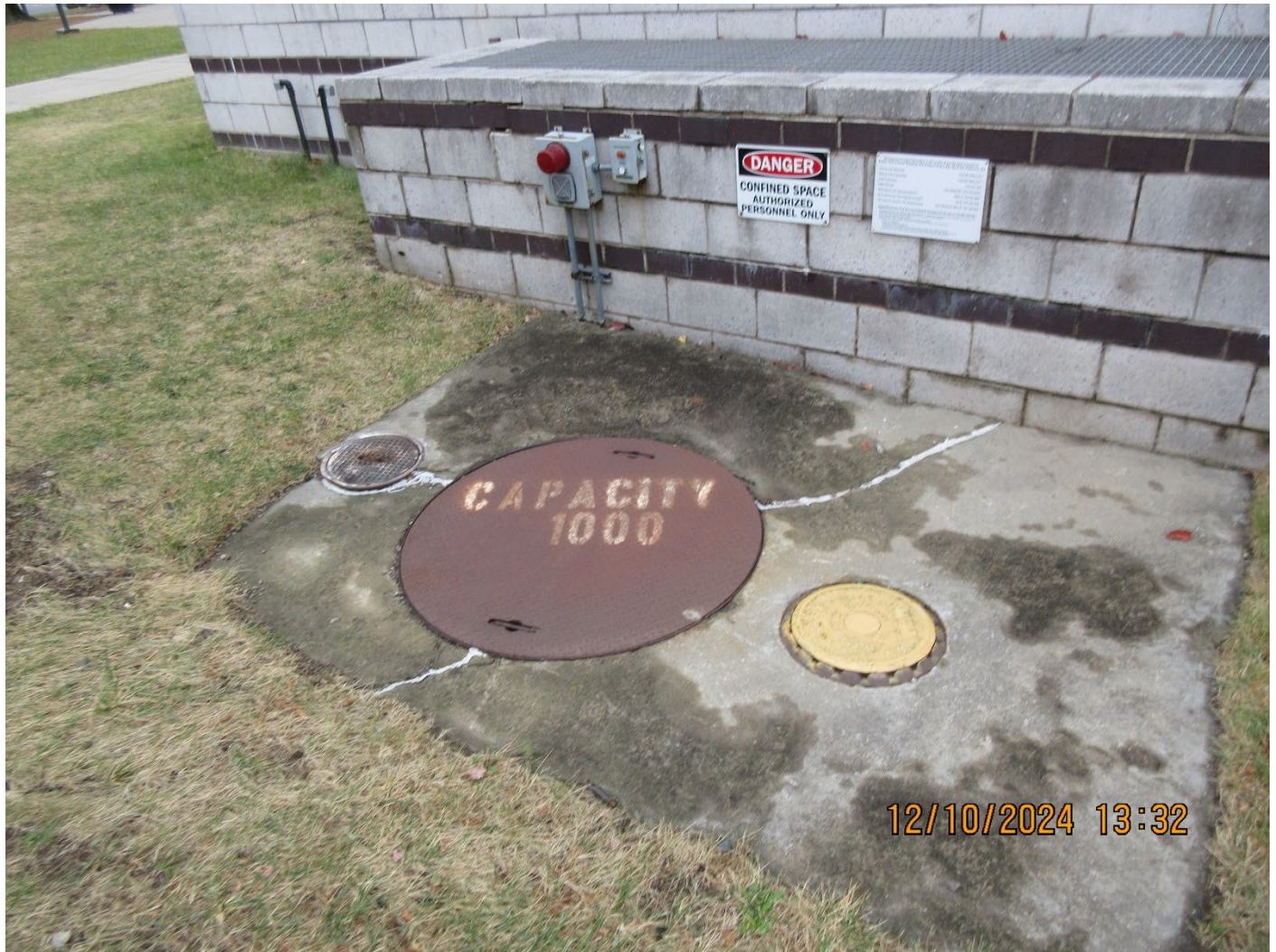
Photo 5 – Exterior photograph of the sumps and access ports along Ward Street.
