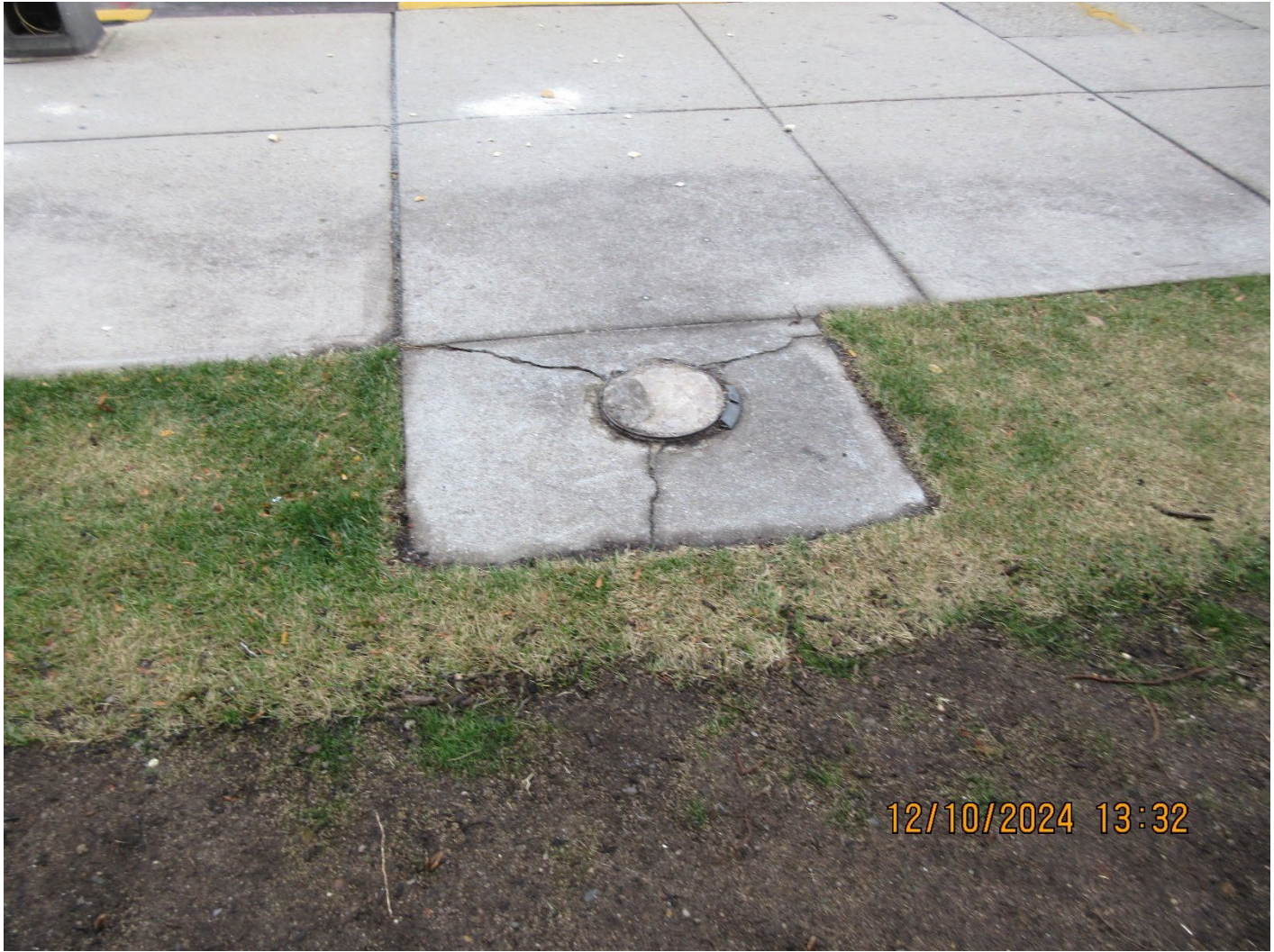
Photo 6 – Exterior photograph of the disused fill port for a previous UST.
