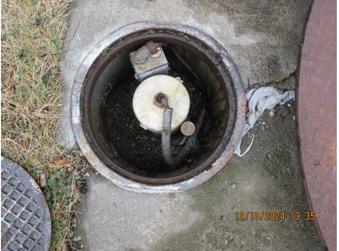
Photo 10 – Annular space access port from above.
