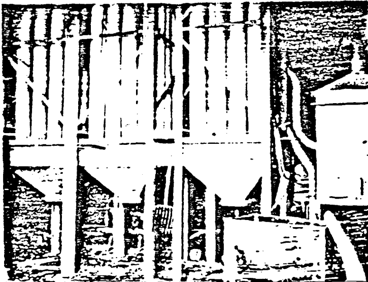
Scrap cutter hood and dust collector
