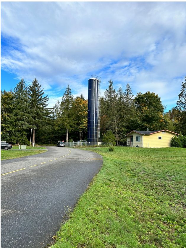
Water Storage Tank
