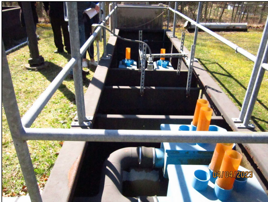
Photograph 16. IMG_0049.JPEG View, facing south, of the CCC. A V-notch effluent weir was present on the south end.
