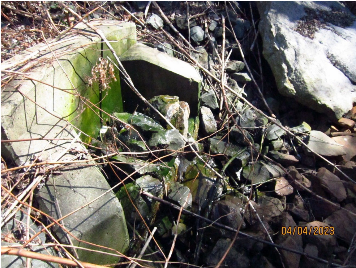
Photograph 19. IMG_0062.JPEG View of Outfall 001 and riprap with algal growth.
