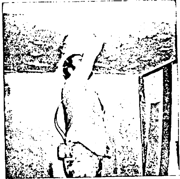
4 (b) Sanding ceiling tape-joints
