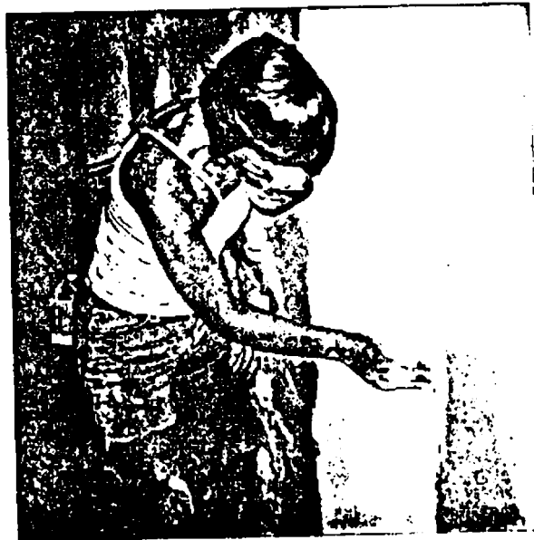
5 (c) Sanding wall joints
