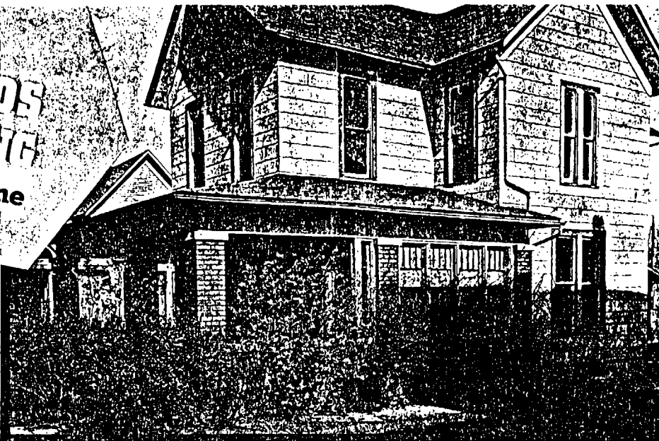
USG No. 600 Wavy Butt Siding was used to transform the house at the left to the fine-looking home you see above. In addition to improving the appearance of the home, USG Asbestos Cement Siding gives added protection from fire and weather, helps make the home more comfortable summer and winter.
