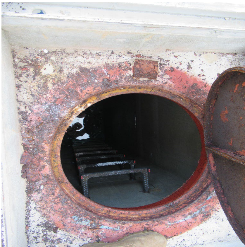
Photo 41- Bldg. 845; potable water storage tank hatchway (2of 2)
