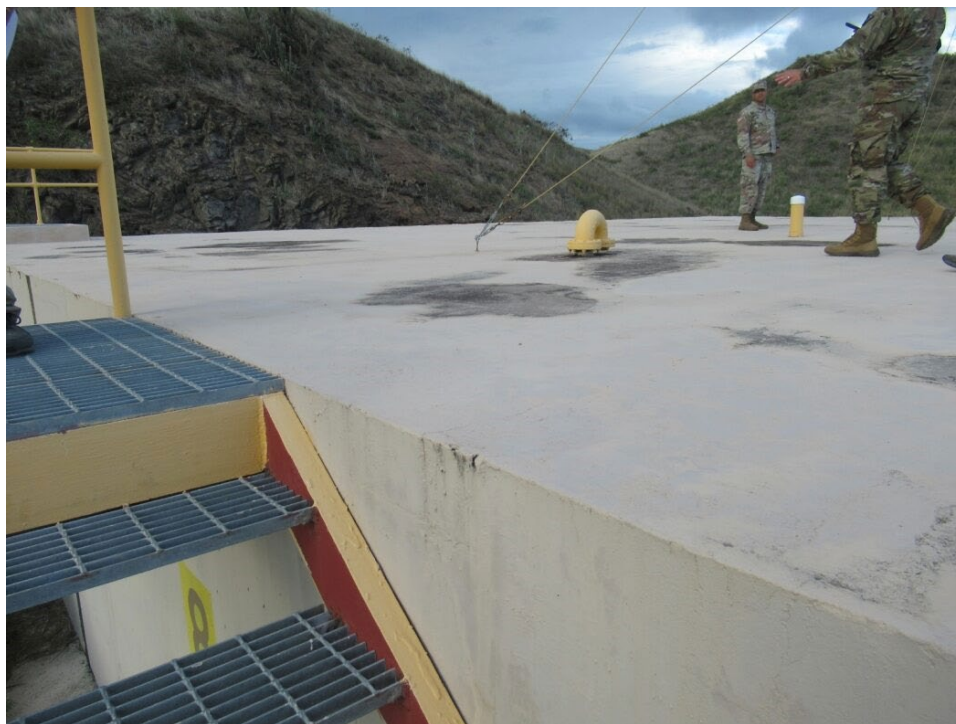
Photo 42 –Bldg. 845; surface of potable water storage tank (1 of 3)
