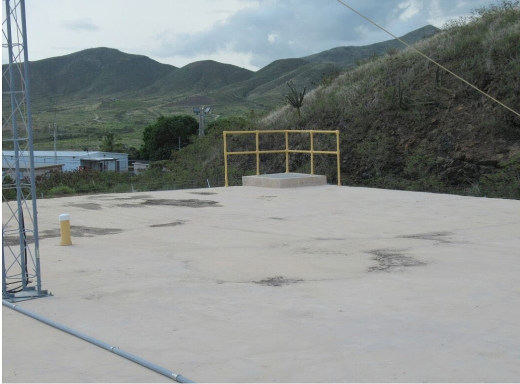
Photo 43 -Bldg. 845; surface of potable water storage tank (2 of 3)
