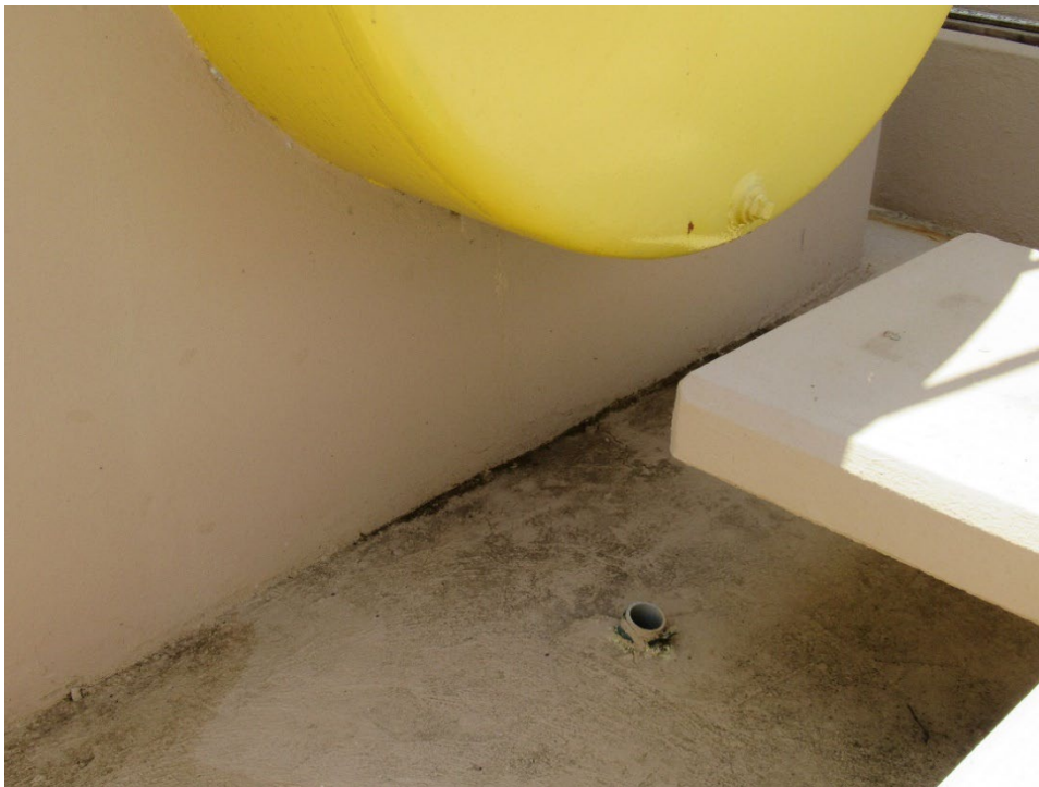
Photo 32 –Bldg. 00341; diesel fuel tank secondary containment; in-ground vertical pipe
