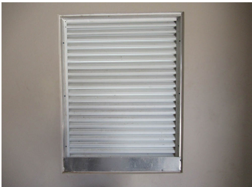
Photo 22 – Chlorine injection building; louvered window
