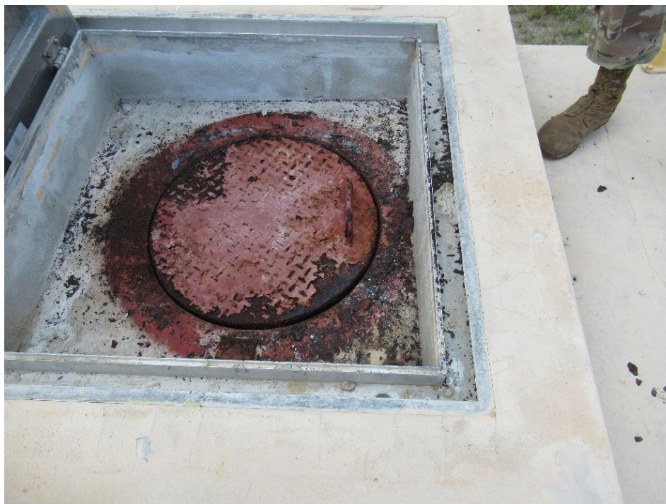
Photo 40 – Bldg. 845; potable water storage tank hatchway (1 of 2)
