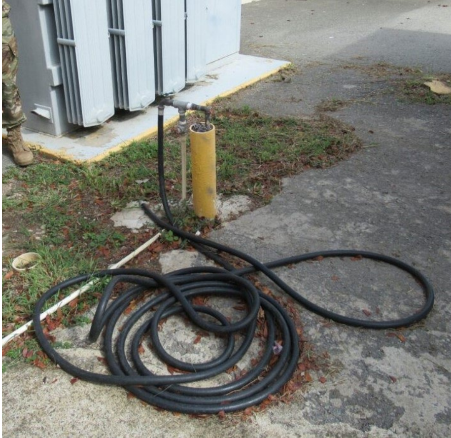
Photo 37 – Bldg. 1011; outdoor faucet with connected hose
