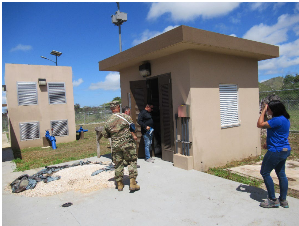
Photo 23 – Chlorine storage shed
