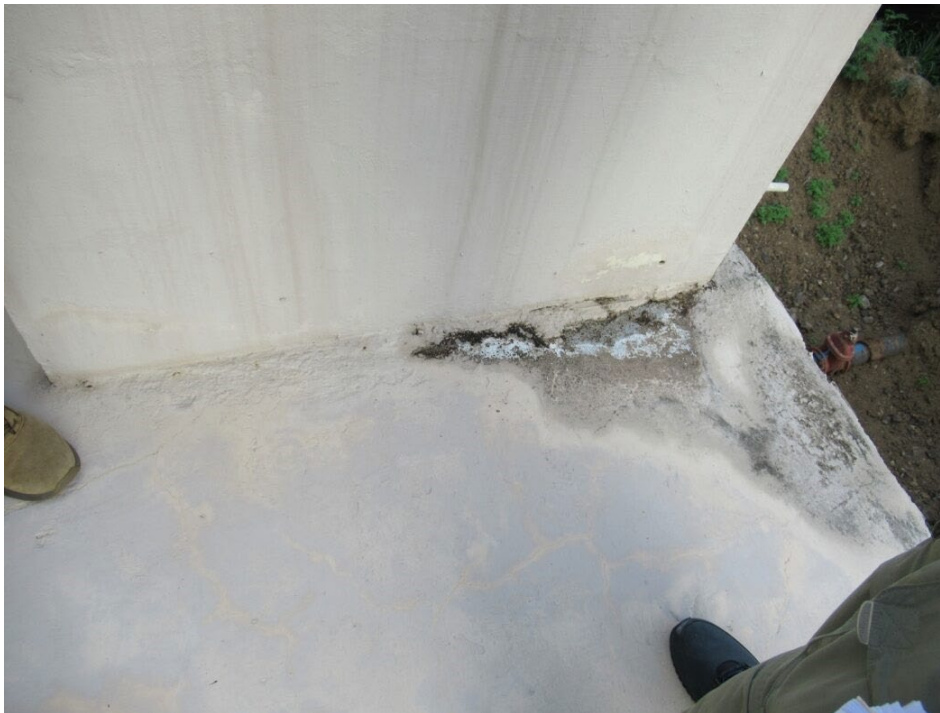
Photo 44 – Bldg. 845; surface of potable water storage tank (3 of 3)
