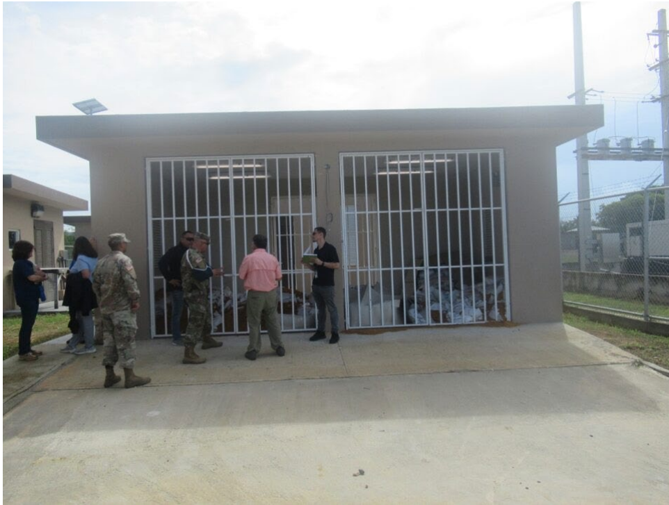
Photo 11 - Shed in Well No.2 enclosure, bags of ion exchange resin
