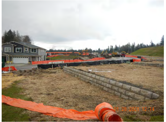
Photo #:18 (DSCN2035) Description: Facing north, photo of the Phase 1 area just east of the main entrance.
