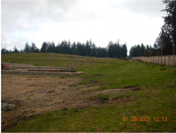
Photo #:17 (DSCN2034) Description: Facing east, photo of the stabilized areas near the southwest corner of the development.
