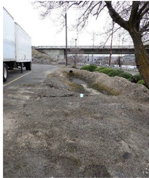
Photo #:20 Description: Facing south, photo of the PL infiltration basin and sampling location.
