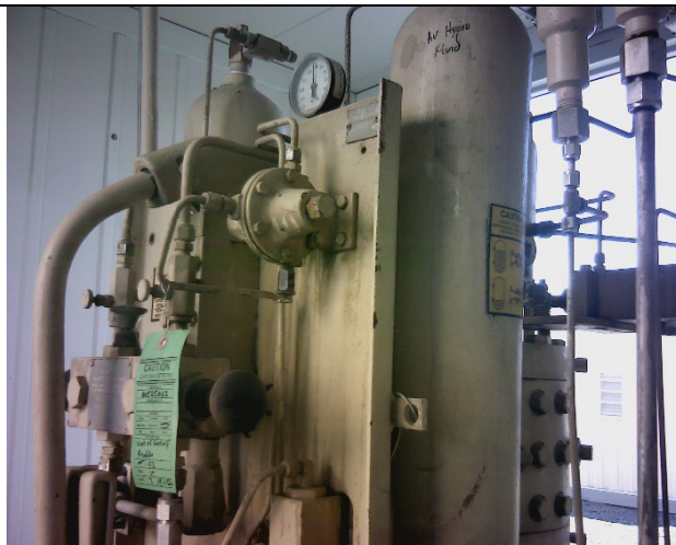
Figure 4: Inside Valve 65 B Shelter. A leak was found on this valve regulator. Montrose tagged the leaking component upon discovery. Tag No. 60525062. Source: Open-Ended Line. This leak was repaired on 8/9/22 according to facility records. (See Attachment 4-D, 7/19/2022 OOOOa Survey Details.)
