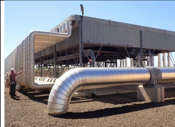
Figure 1: Gas Cooler System. EPA Inspector Heins (foreground) checking for fugitive emissions using a TVA 2020 instrument (Method 21), while EPA Inspector Pavitt (background) uses a FLIR Camera (OGI).
