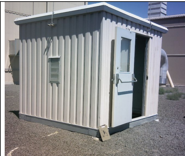
Figure 3: Shelter for Valve 65 B (B-Line Blowdown Valve). One of multiple shelters that are part of the facility's monitoring plan for undergoing quarterly Leak Detection and Repair (LDAR).
