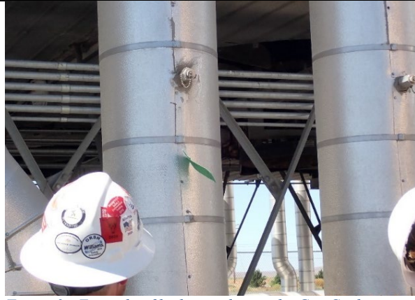
Figure 2: Example of leaking valve on the Gas Cooler found using Method 21. A tag was applied to the location by Montrose. All 11 leaks from the Gas Cooler were repaired by 8/9/22 according to facility records. (See Attachment 5-D, 7/19/2022 OOOOa Survey Details.)
