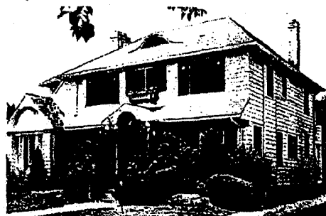
AFTER: See what two coats of SWP accomplished over this weather-worn surface--a rejuvenated house at the cost of only a paint job!
