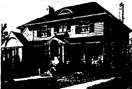
BEFORE: This shingle house was neglected for several years after painting with a hard-drying paint which cracked badly--making a difficult surface to paint properly.
