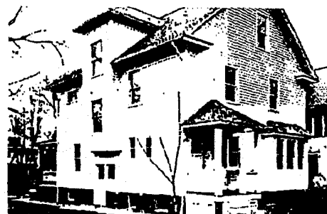
AFTER: One coat of SWP Undercoater No. 450 produced a uniform smooth foundation coat over this variegated surface and made a superior SWP paint job possible.
