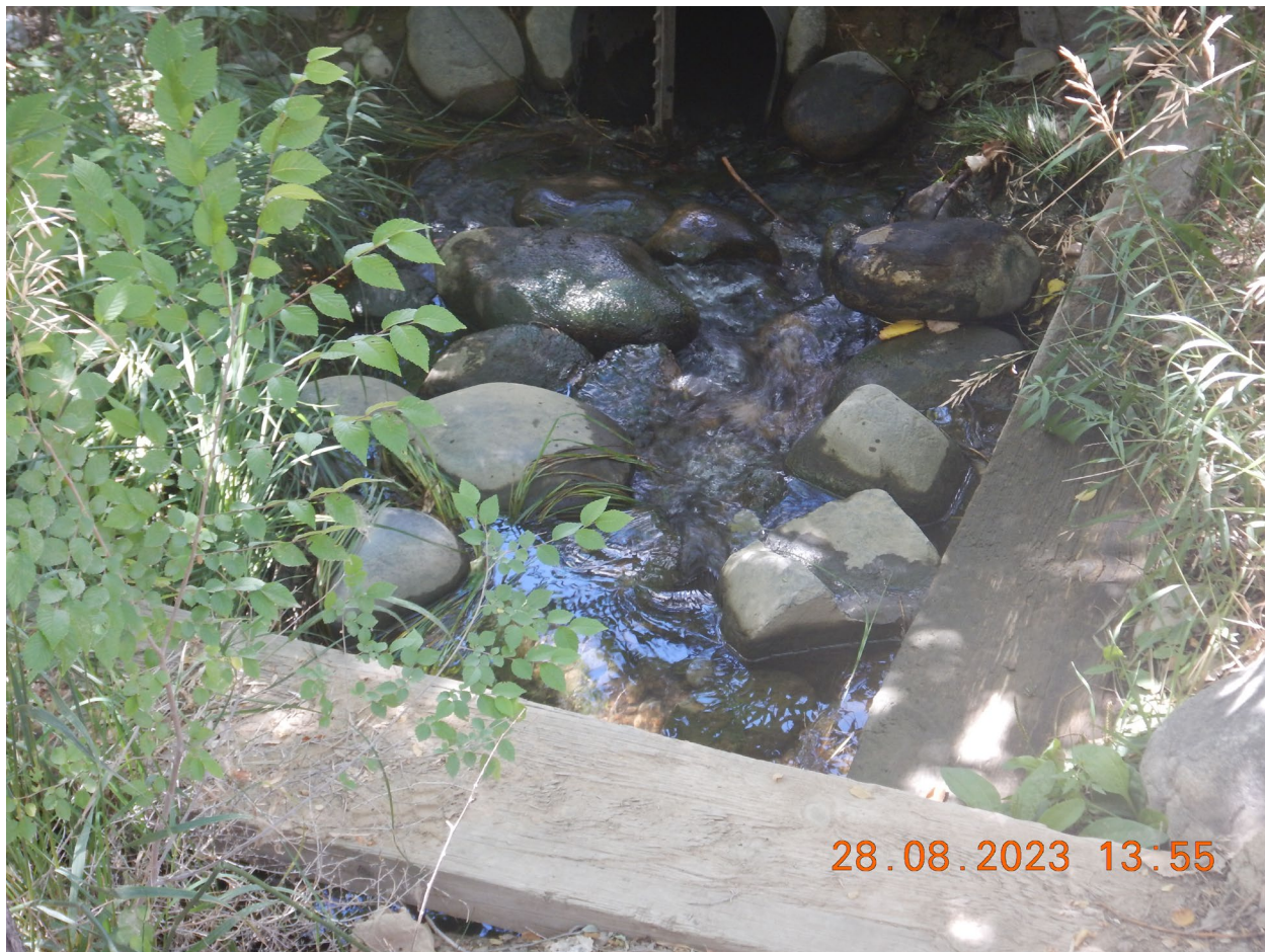
View of the discharge into the open channel, thence into a closed conduit and ultimately into the Lower Animas Ditch. (DSCN2613). Photographed by D. Esparza
