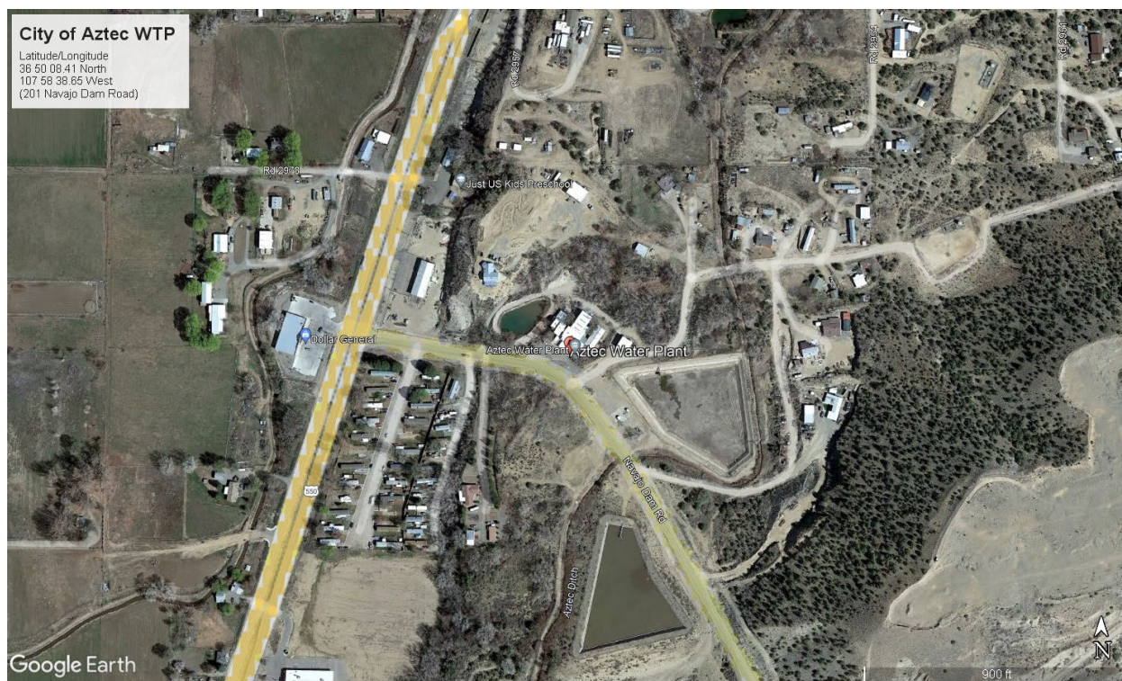
Aerial Image #1 Overall view of the City of Aztec's Water Treatment Plant. Aerial from Google Earth.
