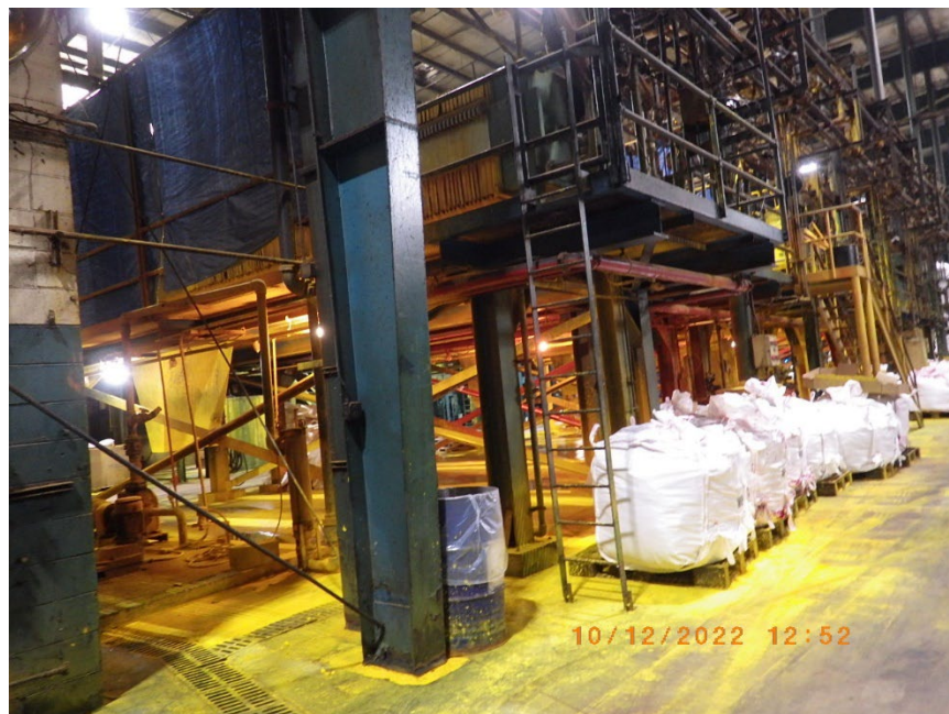
10: APOL0319 Description: Yellow pigment filter presses Location: Northeast side of Building 2 Camera Direction: South Date/Time: 10/12/22, 12:52 p.m.
