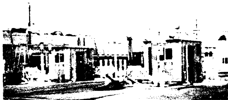
Figure 3 Operator shacks at bottom loading facility
