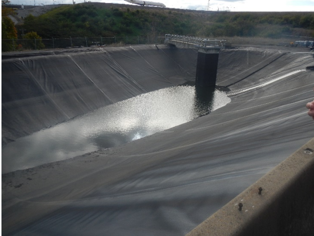
Photo 1. Aerated Lagoon, north section.
