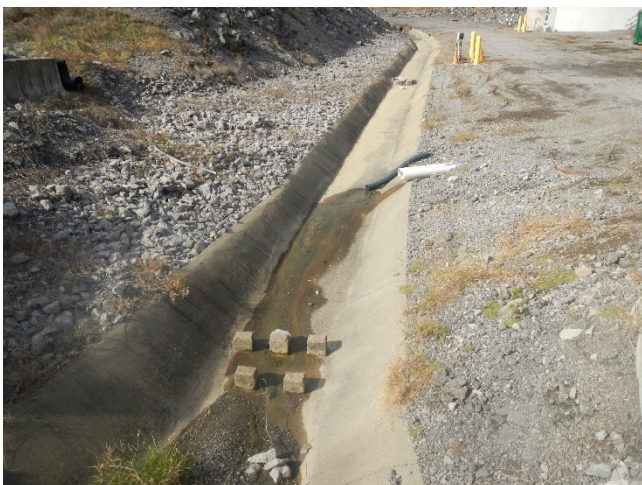
Photo 5. Open channel ditch from the Clarifier (in the background) to Sims Creek/Outfall 002.
