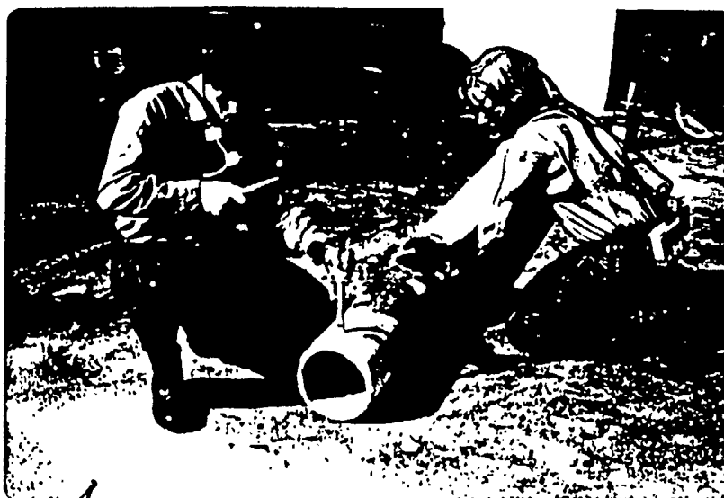
FIGURE 9. Cutting pipe with hammer and chisel.
