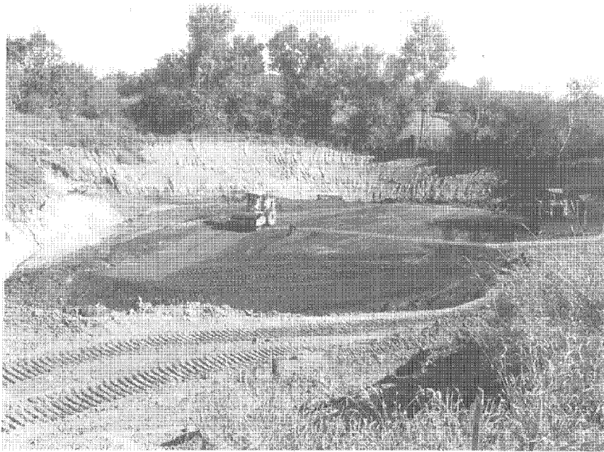
• Photograph 46: Backfill and Compaction.
