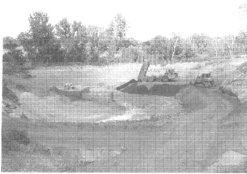
• Photograph 45: Backfilling.
