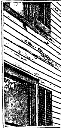
In this siding can be noted paint peeling from the boards as the result of moisture back of the paint
