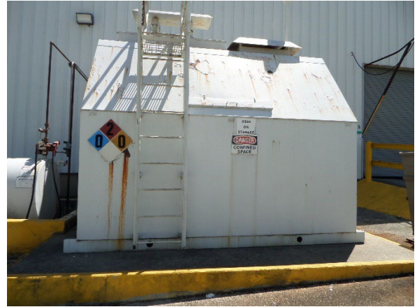
Photo-4 4000-gallon Used Oil Tank
