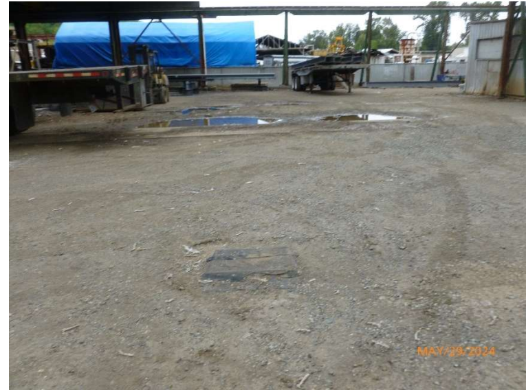
Photo 10: P101580 05/29/2024 Southern Stormwater Catch Basin with Filtration BMP – Directly East of North End Of Canopied Work Area
