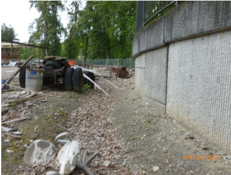
Photo 9: P1010579 05/29/2024 Drainage Swale Along Facility-Green River Trail Structure Border (looking north)
