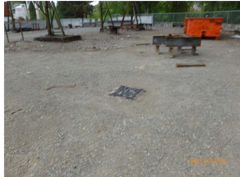
Photo 12: P1010582 05/29/2024 Northern Stormwater Catch Basin with Filtration BMP – Looking North toward Facility's Entrance/Exit to South 143 rd Street
