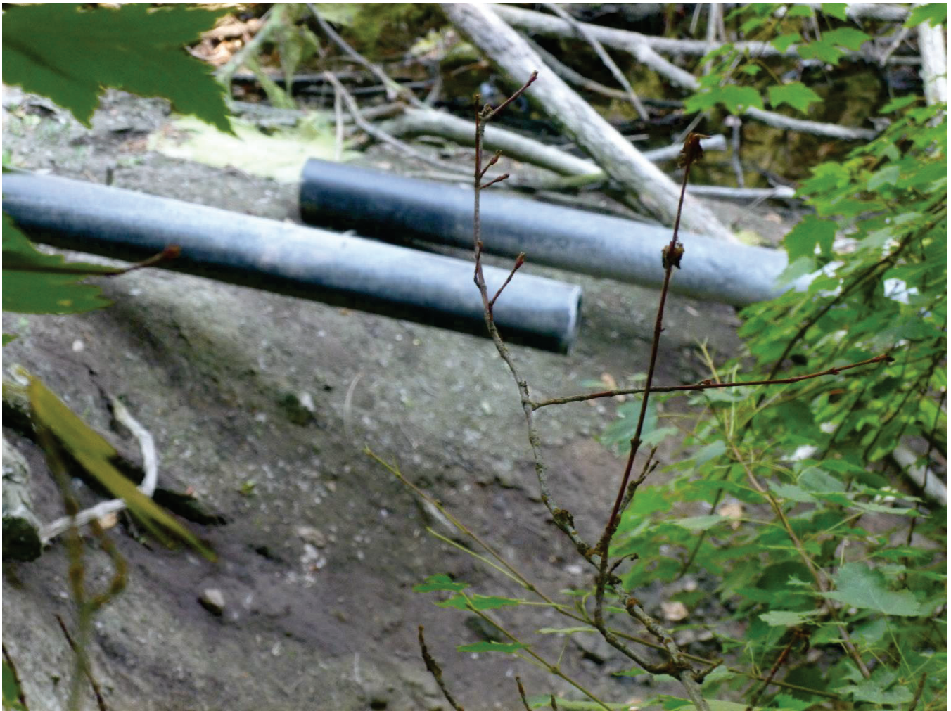
Photo 2 / P1000998 – Discharge Point 004, close up
