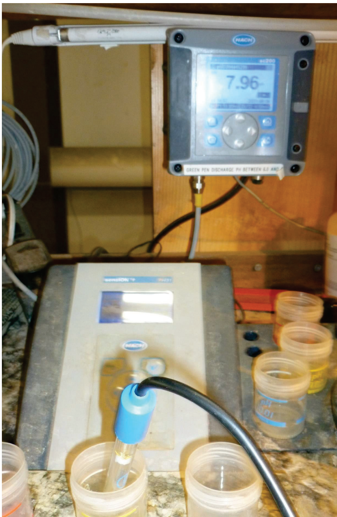
Photo 11 / P1010005 – pH Readout and Control Station
