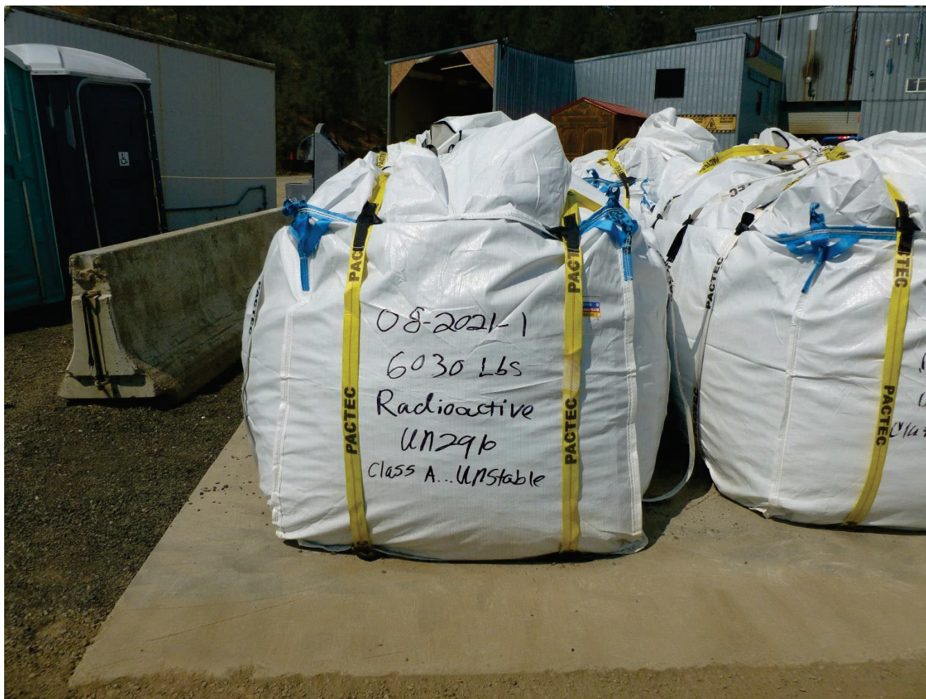
Photo 3 / P1000999 – Totes of Sludge, awaiting transport to processing facility
