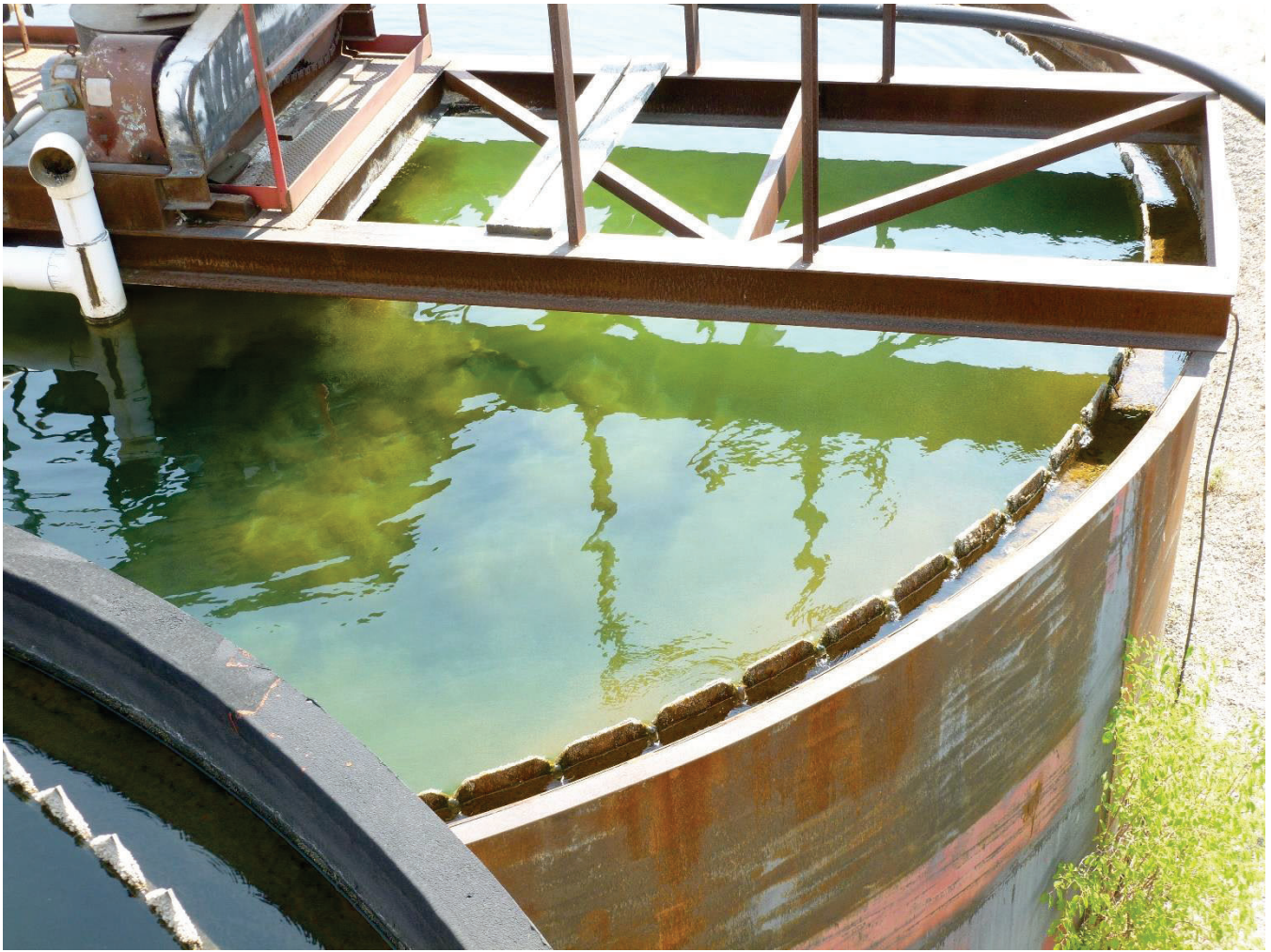
Photo 7 / P1010010 – Wastewater Plant Clarifier, close up
