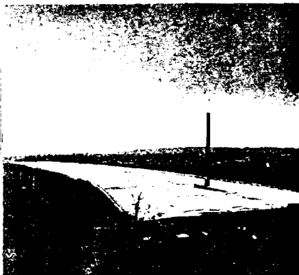
Another view of the Route 80 bridge. Nearly 80 tons of red lead were used to prime the structural steel of this bridge. Superstructure: American Bridge Div., U.S. Steel Corp. Substructure: Conduit & Foundation Corp. (at left)
