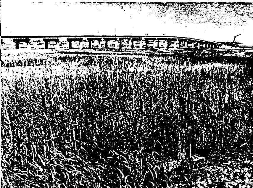
5,000 gallons of red lead paint were used to prime the steel of the Route 3 bridge (shown here and on the cover). It is the first in northern New Jersey to be equipped with low-level fluorescent lights. Superstructure: Phoenix Bridge Co. Substructure: J. Rich Steers Inc.
