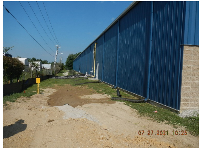
Photo 10: Construction zone SE corner of the building.
