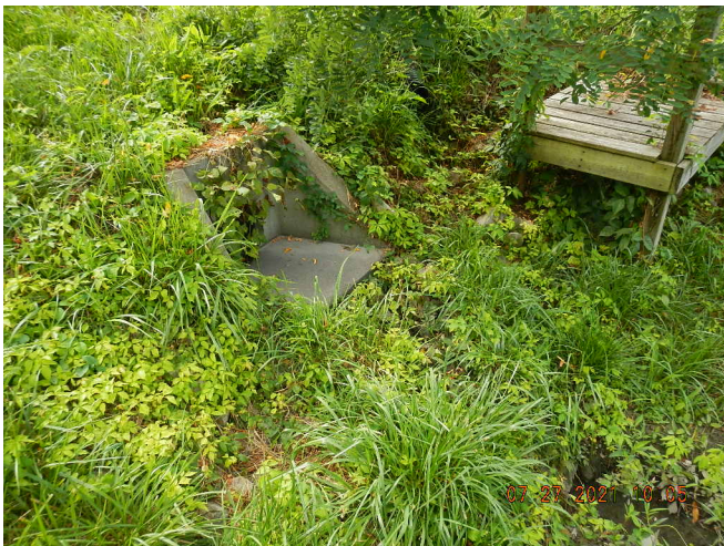
Photo 7: Outfall 001 located approximately 25 feet from the fence shown in Photo 8.
