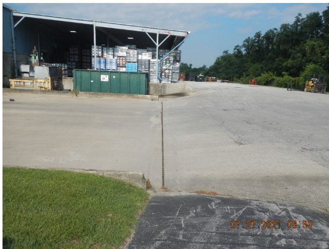
Photo 1: Loading dock drainage and truck loading garage. N-NE side of the building.
