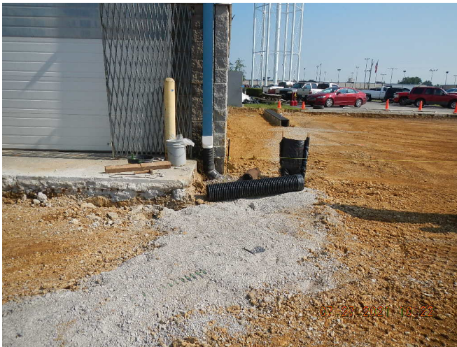
Photo 9: Construction zone SE corner of the building.
