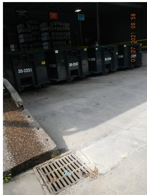
Photo 2: Loading area storm drainage. N-NW side of the building.
