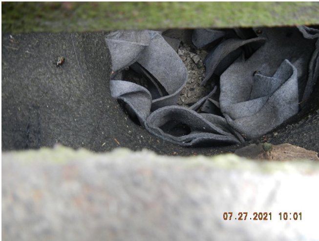
Photo 3: Loading area storm drain sock to catch gravel and other solids inside the culvert shown in Photo 2.
