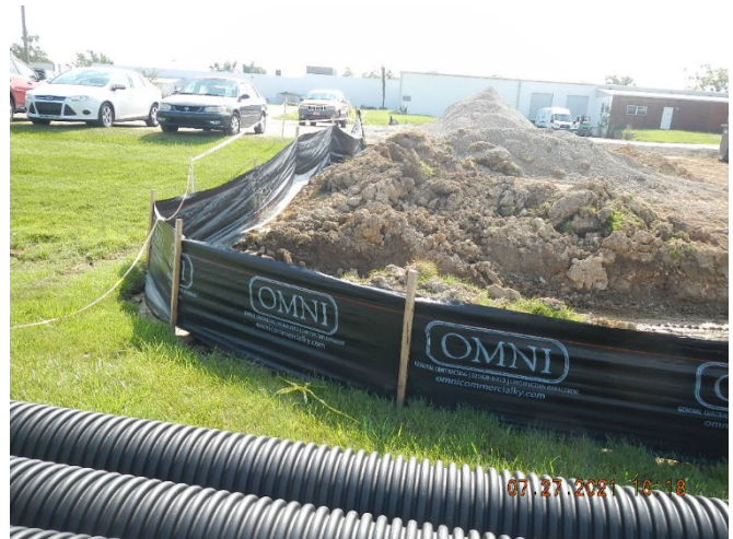
Photo 8: Construction zone silt fence. East side of the building.
