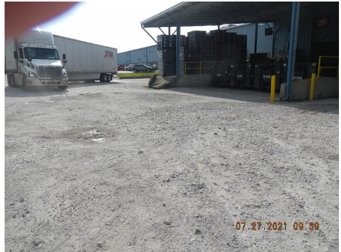
Photo 4: Gravel lot. N-NW side of the building.
