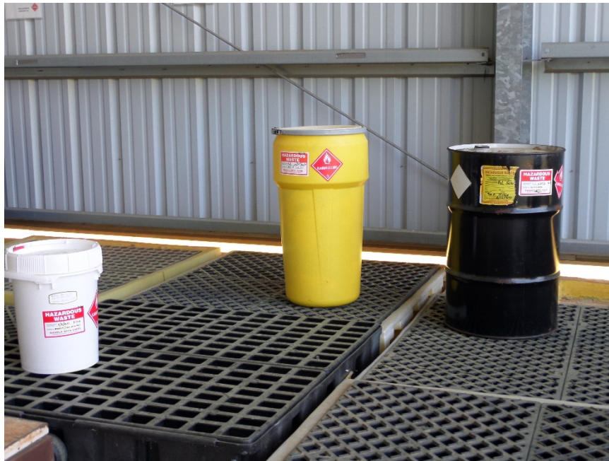
Photograph 3: Hazardous waste containers in the facility's hazardous waste central accumulation area.
