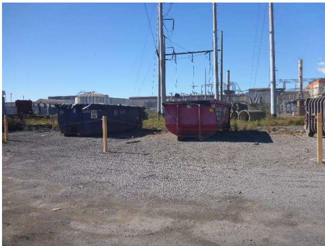
Photo 16: East of EAF Baghouse – Storage Pad
