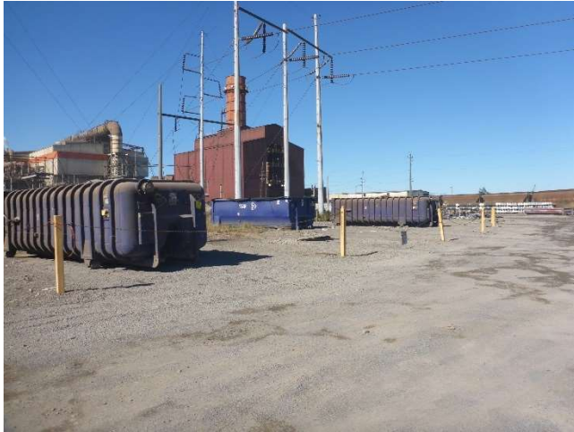
Photo 15: East of EAF Baghouse – Storage Pad
