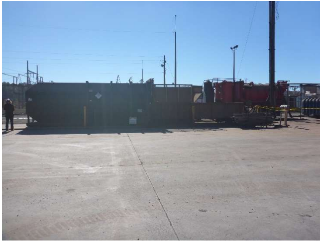
Photo 13: East of EAF Baghouse – Compactor
