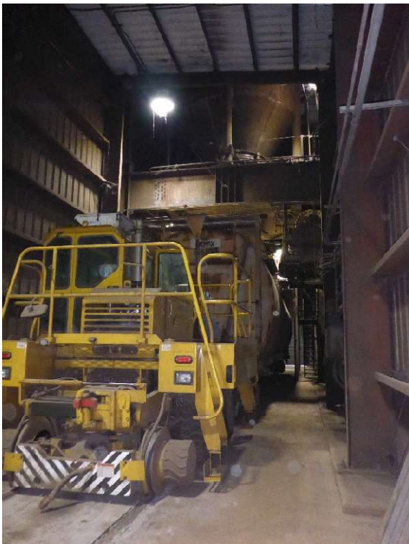
Photo 26: EAF Baghouse - Loadout Building
