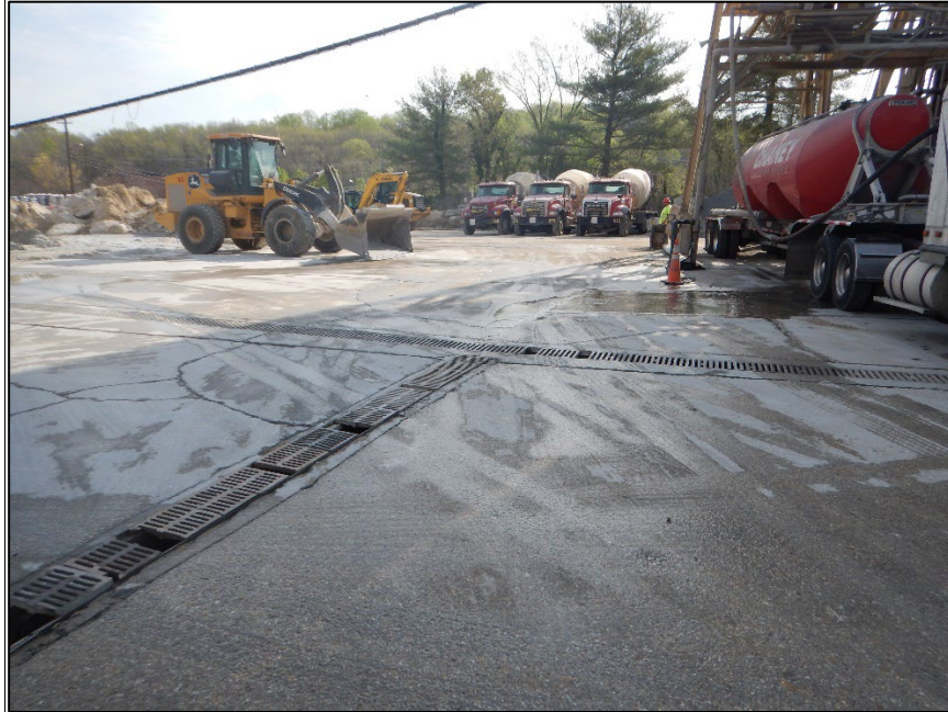
Photograph 1. DSCN8728.JPEG View of central portion of the Facility. Note the trench drains bisecting the area.
