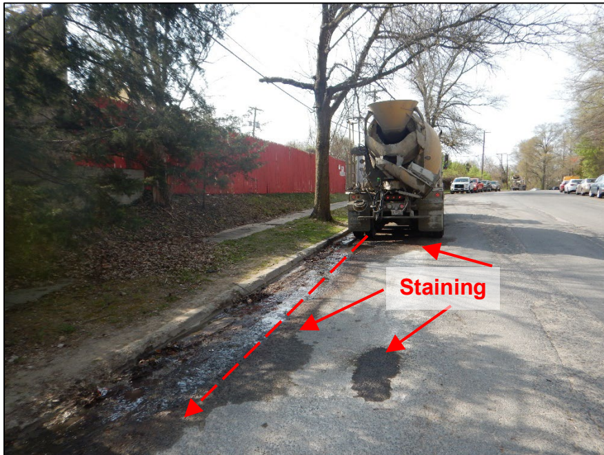
Photograph 10. DSCN8758.JPEG View, facing south, of flow from Outfall 002 in the curblines along Chrysler Way. Note the truck queued in line for the Facility along the public road. Some petroleum product staining was present in and near the curblines.
