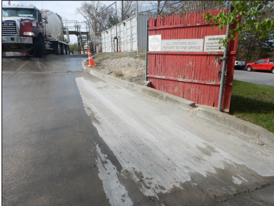
Photograph 19. DSCN8789.JPEG View of sediment track-out downgradient of the wash area trench drain.
