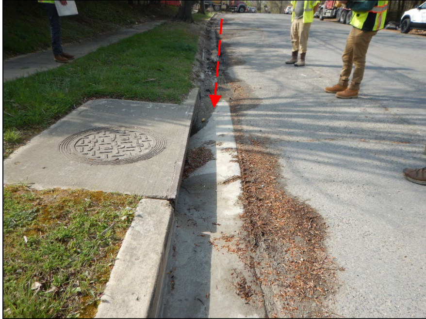
Photograph 11. DSCN8760.JPEG View, facing south, of flow from Outfall 002 in the curbline along Chrysler Way, entering the county storm sewer inlet.
