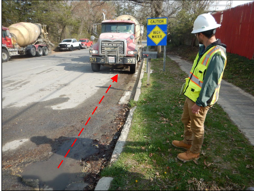
Photograph 9. DSCN8755.JPEG View, facing north, of flow from Outfall 002 in the curblines along Chrysler Way. Note the truck queued in line along the public road. Sediment and debris were observed in the flow path along the public roadway.
