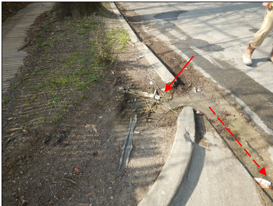
Photograph 8. DSCN8751.JPEG View of Outfall 002 into the curblin along Chrysler Way (white PVC pipe).
