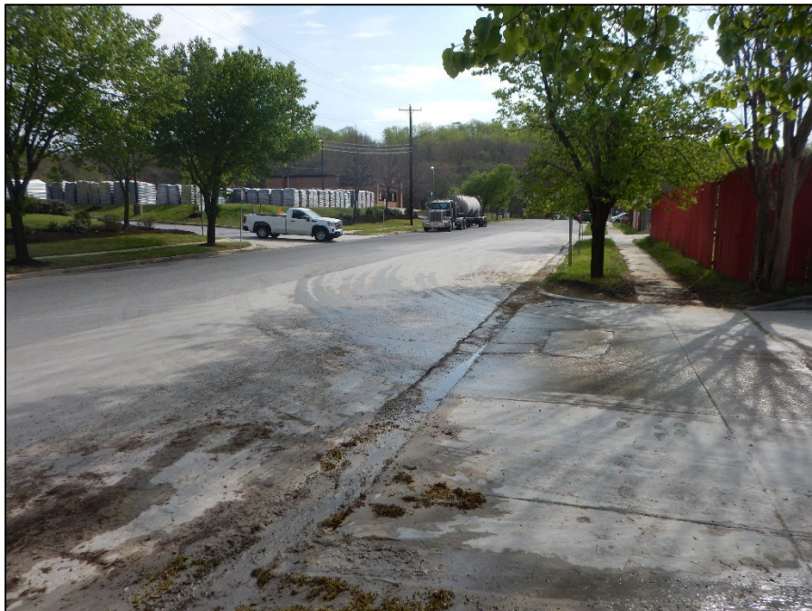
Photograph 20. DSCN8791.JPEG View of track-out and vegetative debris outside of northern gate, near the wash station.
