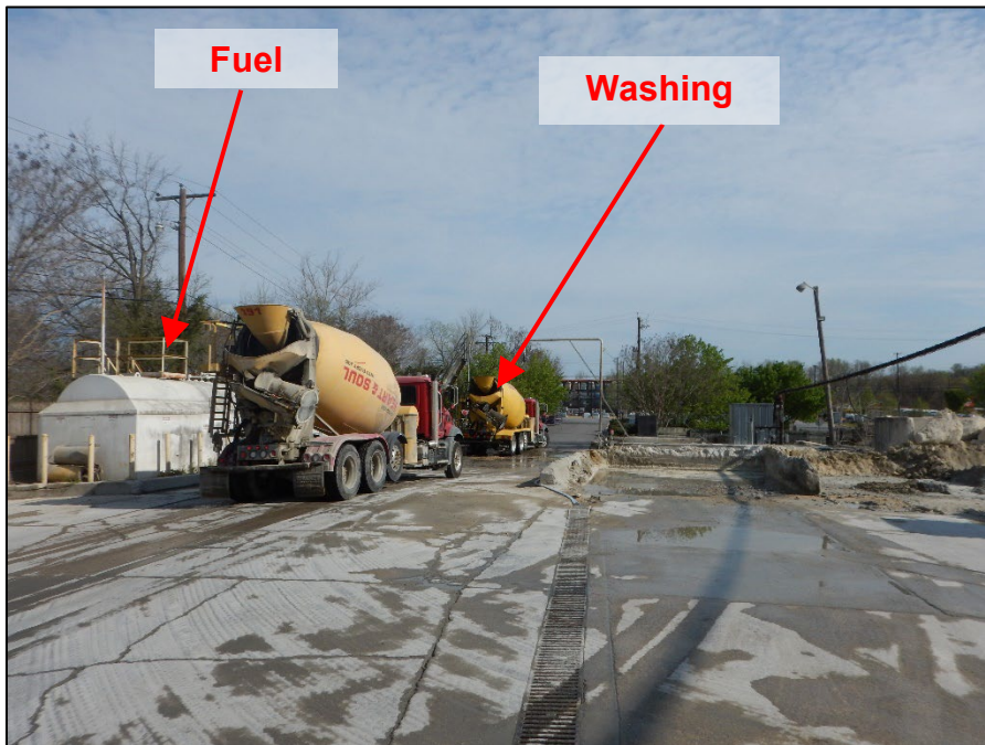
Photograph 2. DSCN8730.JPEG View, facing north, of the fueling and washing stations.
