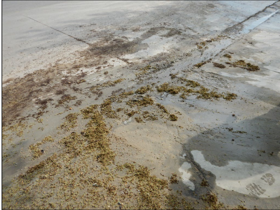
Photograph 21. DSCN8790.JPEG Close-up view of track-out and vegetative debris outside of northern gate, near the wash station.
