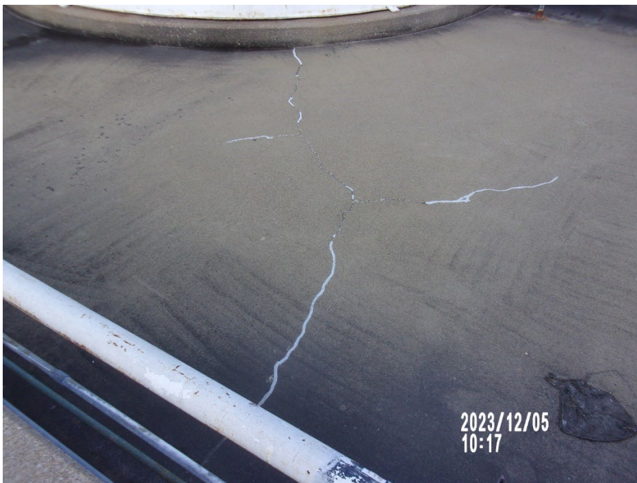
Photo 9: Partially repaired cracks in the secondary containment concrete.
