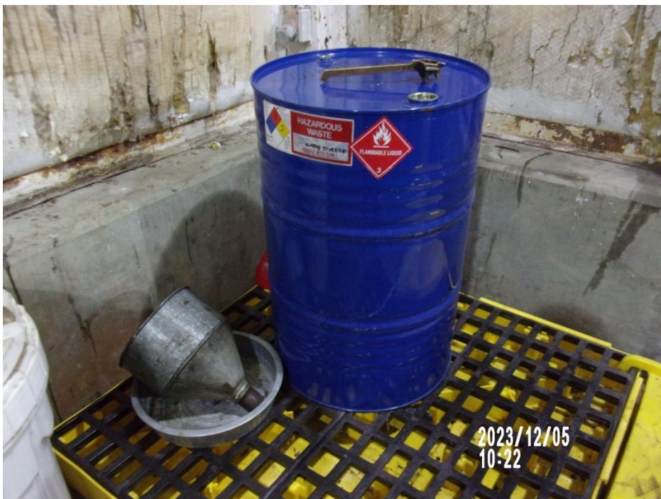
Photo 10: Hazardous Waste SAA Metal 55-Gallon Container in the Pump House.
