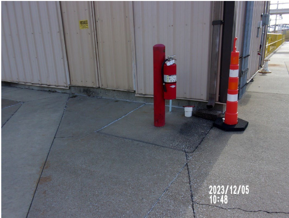
Photo 19: Example Photo of Fire Extinguisher. Fire Extinguishers were present throughout the facility.
