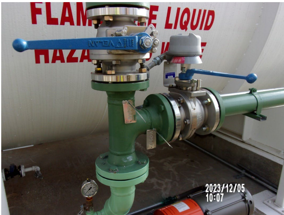
Photo 2: Air Monitoring Tags on the Hazardous Waste Pump Ancillary Equipment.
