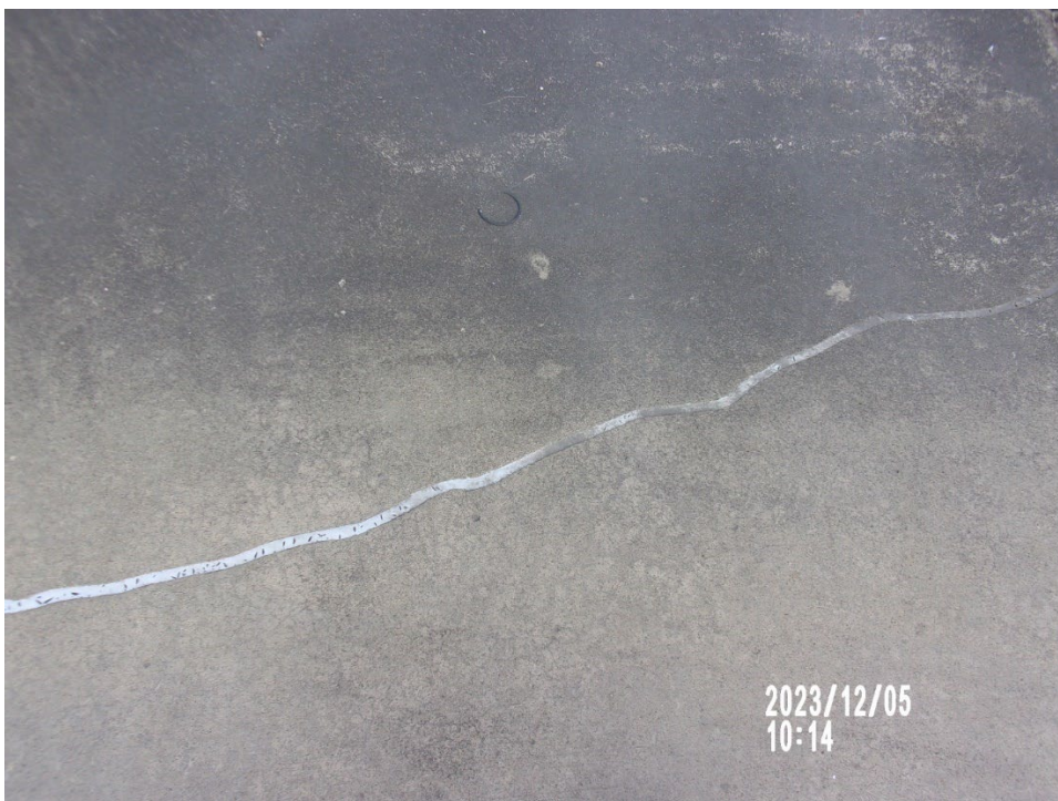
Photo 5: Repaired crack in the secondary containment in the vicinity of the hazardous waste accumulation tank.
