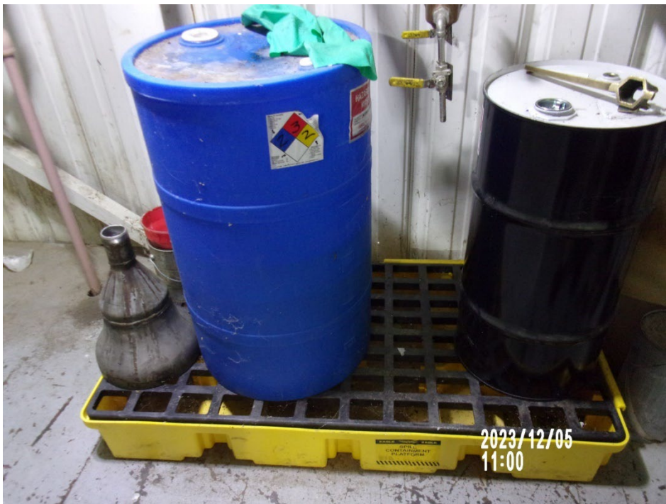
Photo 25: SAA Containers in Plant 1 Containing Waste Initiator and Waste Polymer.
