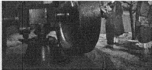
Ten-ton wheels, used to grind black powder, are still in place in mill near Brandywine.
