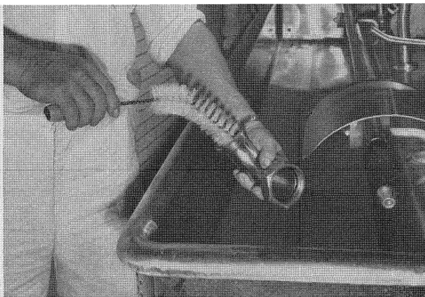
Pipe elbow brush cleans tubes at Wisconsin's Hiawatha Valley Dairies Co-op. Nylon-bristled brushes absorb almost no water, stay sanitary.
