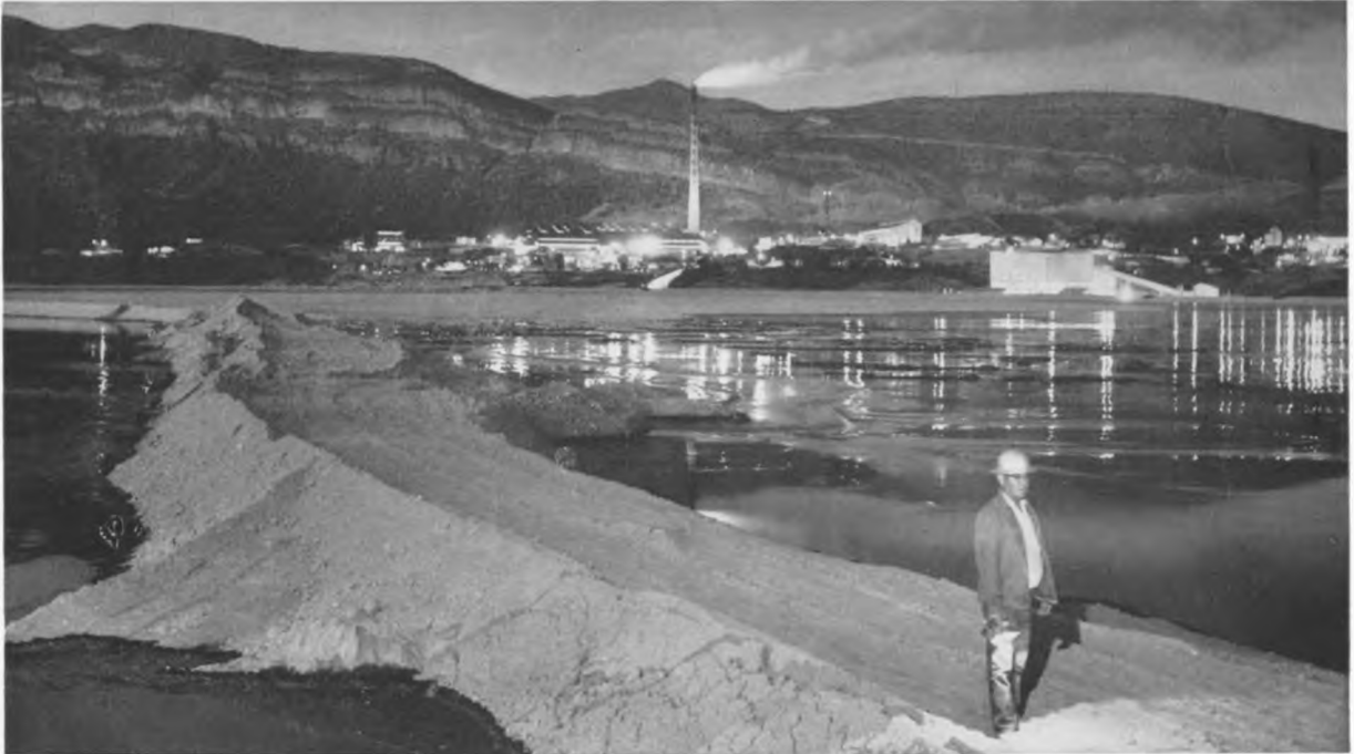
Disposal of waste tailings (the powdered material from which the copper has been extracted) is a problem of major magnitude. The tailings are disposed of by pumping them into "ponds," which are veritable lakes. The photograph above is of the tailings pond at our Ray Division in Arizona.
